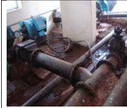
Old pump needs to be replaced
