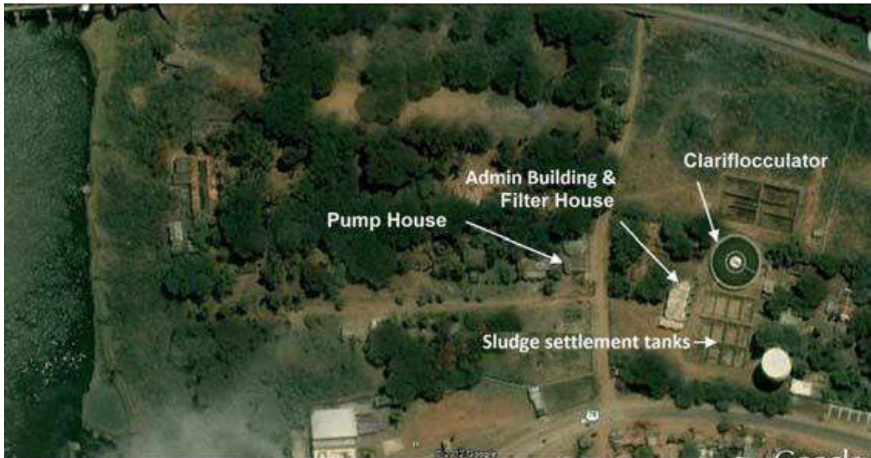
Figure 5: View of Existing WTP components
