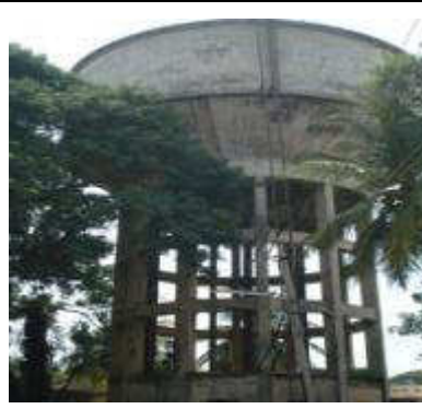
Court Tank to be repaired
