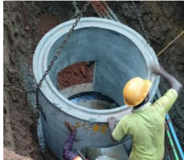
Partial compliance – use of personal protective equipment at Davangere
