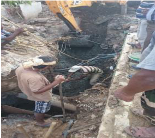
Partial compliance – use of personal protective equipment at Davangere
