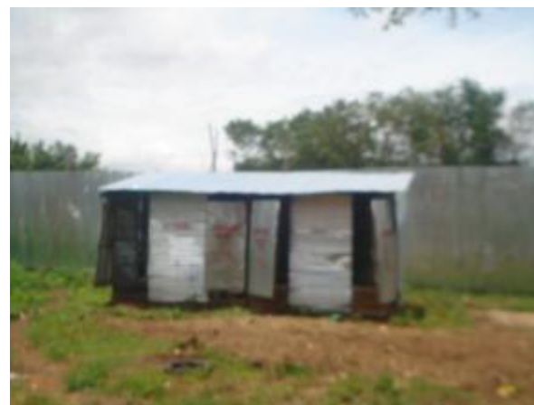
Toilet facility within labour camp at Harihar
