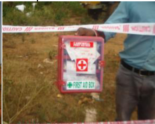
First aid box at one pipe laying location – noted at Harihar
