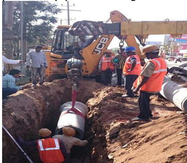
Pipe laying done –Davangere project site.
