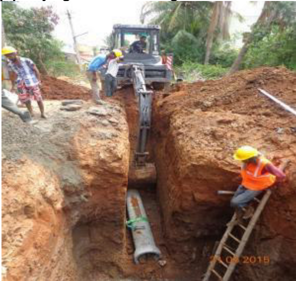
Partial compliance – use of Personal protective equipment
