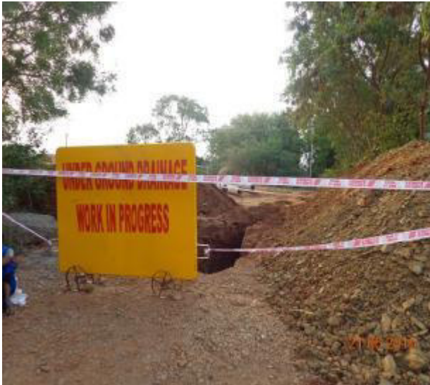
Caution tape and barricade noted at pipelaying area of Davangere
