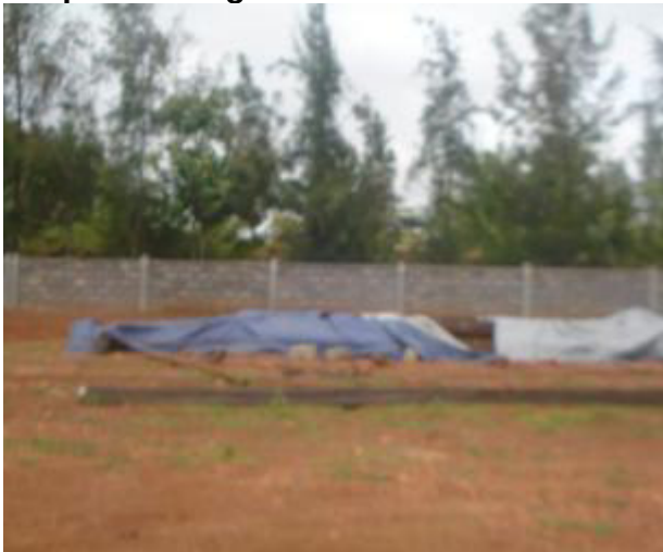
Use of cover for storage of materials
