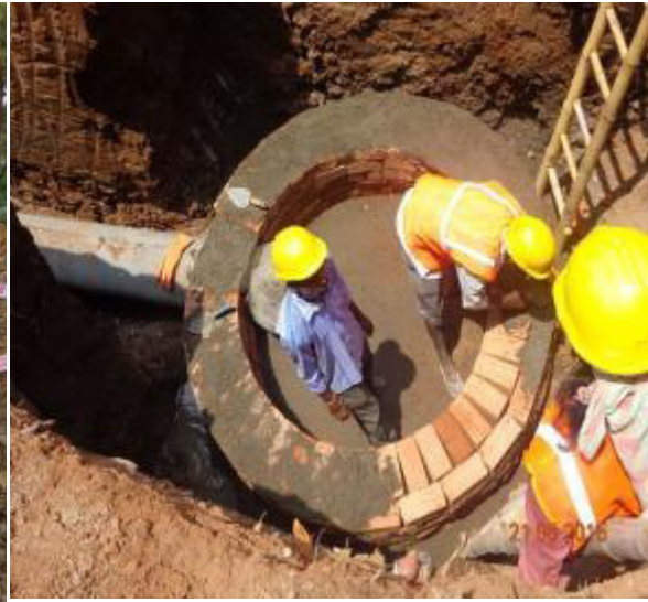
Partial compliance – use of Personal protective equipment
