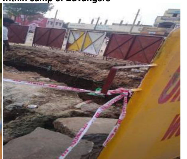
Barricading at pipe laying area of Davangere
