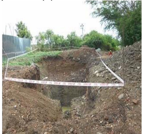
Temporary arrangement of caution tape at excavated area of pumping station. No hard and permanent barricade noted
