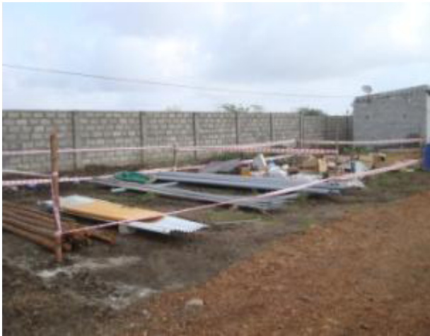
Storage of scrap materials – proper demarcation
