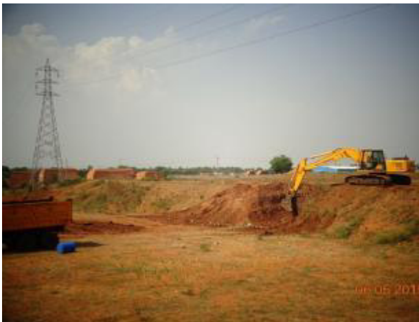
Excavation of bunds at STP site just started
