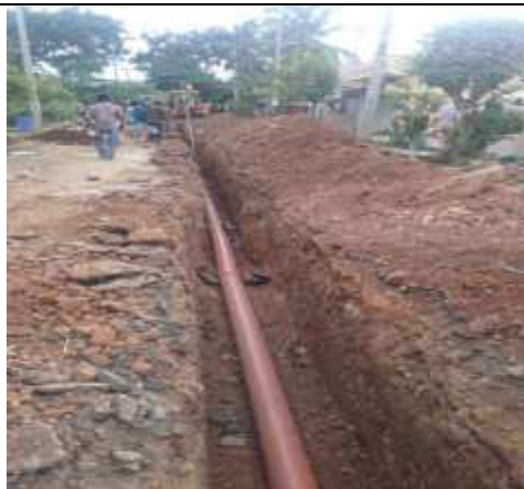
UPVC pipe laying
