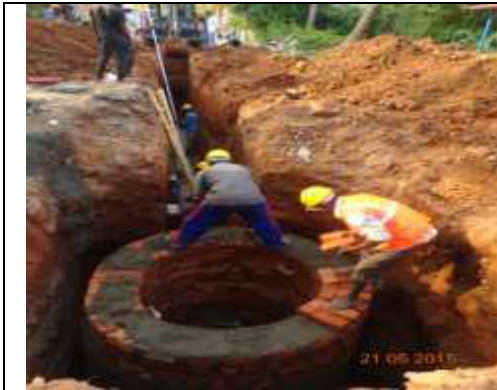
Construction of brick masonry manhole
