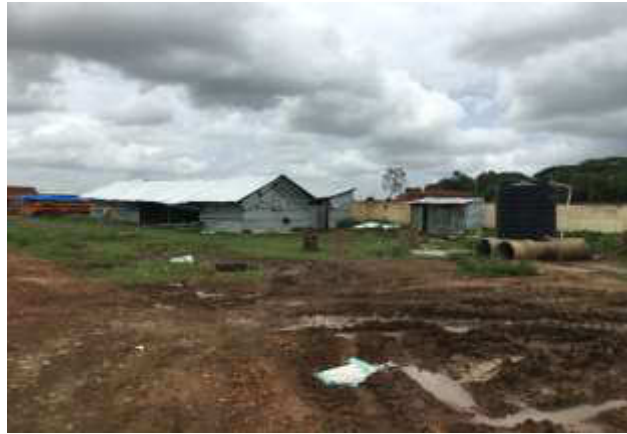
Labour camps at construction site
