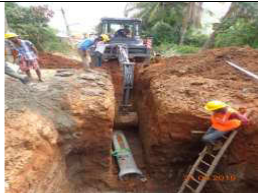
Excavation for RCC pipe laying
