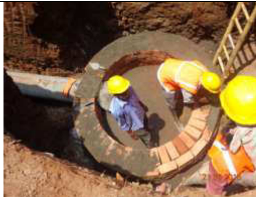
RCC pipe laying
