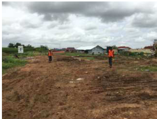
Workers at site
