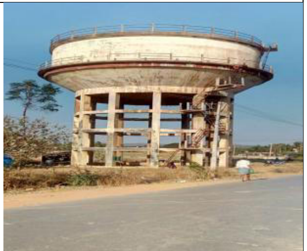
Gandhi Nagara OHT- existing water
