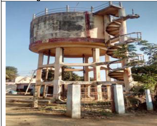
Agasanahalli OHT- existing water reservoir
