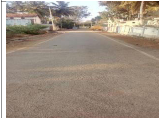
Nehru Nagar area – Water distribution area
