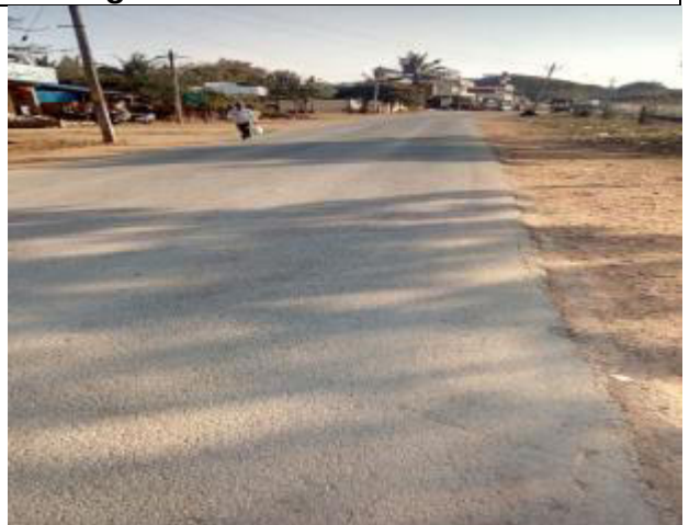
Rattihalli Road- Water distribution area
