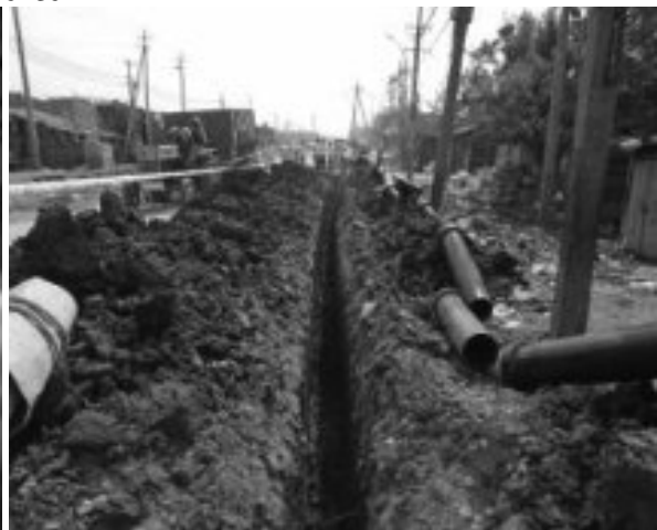
Caution tape at pipe laying area of Davangere. Removal of excess earth is required
