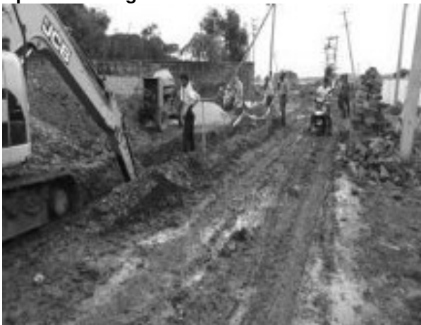
Movement of vehicle during monsoon at pipe laying area at Harihar. Working area demarcated by flags and caution tape
