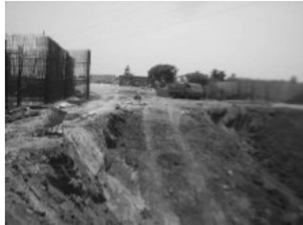
No caution tape at excavated area – 5 MLD STP at Avaragere
