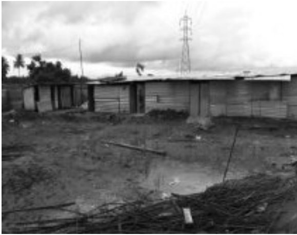
Toilet needs to be improve at 5 MLD STP site
