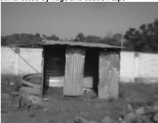
Incomplete toilet facility for labourers at STP site of Harihar
