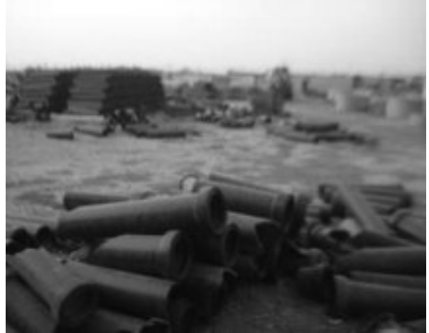
Improper storage of pipes
