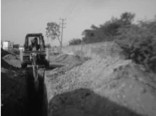
Excavation work is going on for pipe laying
