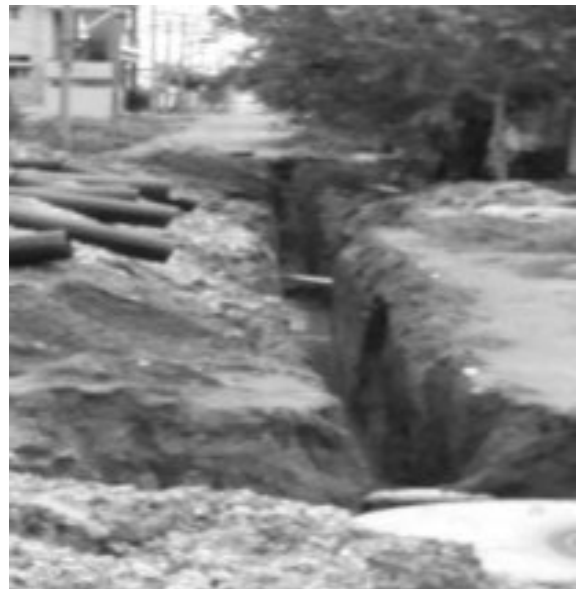
No caution board or display board at working area
