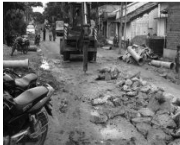
Operation of concrete breaker. Generation of high level of noise. No use of ear plugs by operator
