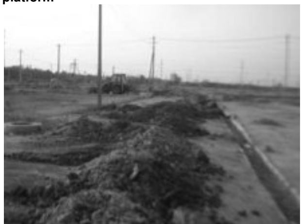
Excess earth after pipe laying- needs to be remove
