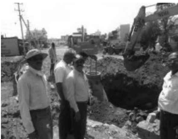
Interconnection work going on at Davangere
