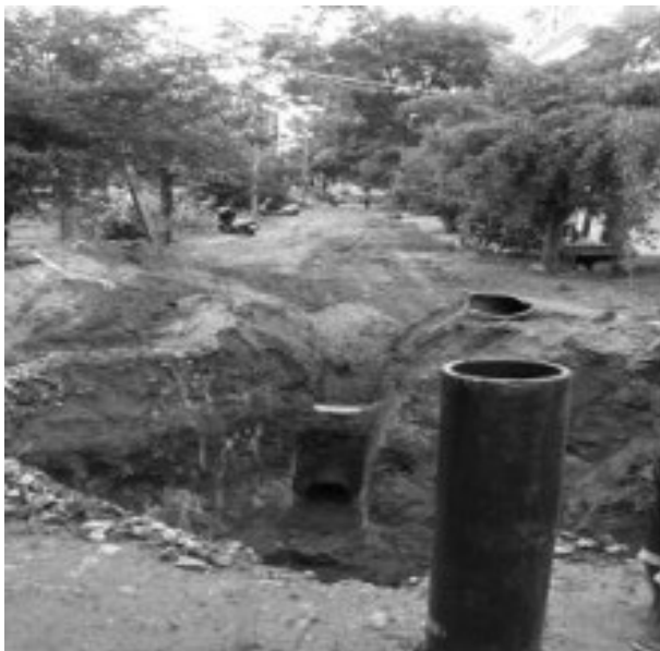
Pipe laying work continued at Davangere
