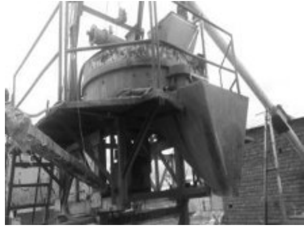
Batching plant at STP- Consent from Pollution Control Board obtained
