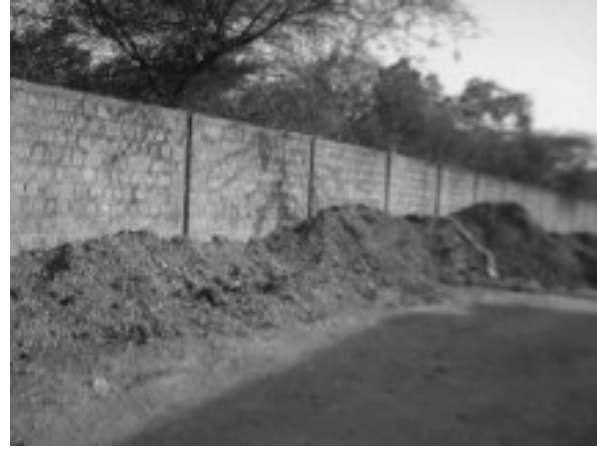
Overburden earth needs to be dispose from working site
