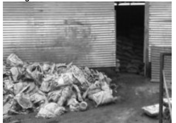
Proper storage of cement within closed room. Disposal of cement bag is required
