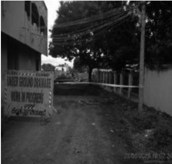
Road closure – display board and caution tape at working location of Harihar
