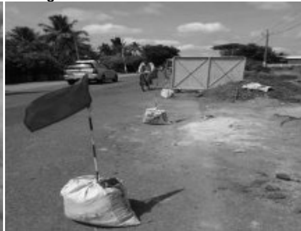
Demarcation of construction area by red flags and board noted at Harihar
