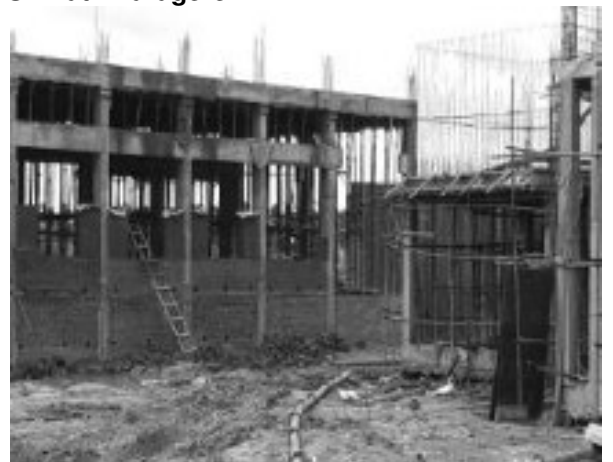
Construction going on for 20 MLD STP at Davangere
