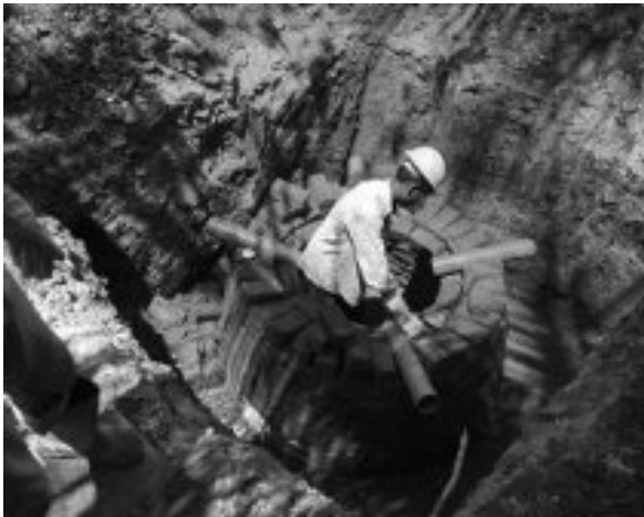
Use of PPE by worker for pipe laying work at Harihar
