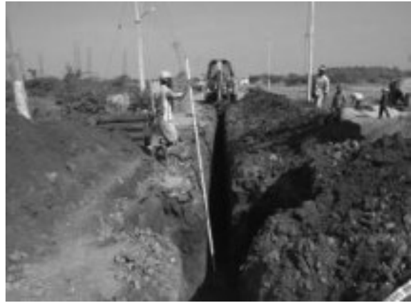
No caution tape at working area
