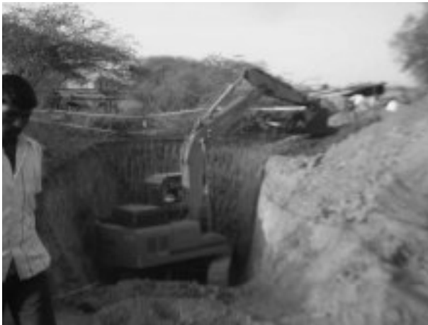
Excavation work going on for lifting station at APMC. Incomplete arrangement of caution tape and no hard barricading at construction site
