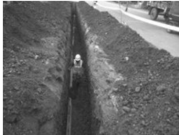
Partial use of PPE by worker- no proper shoes
