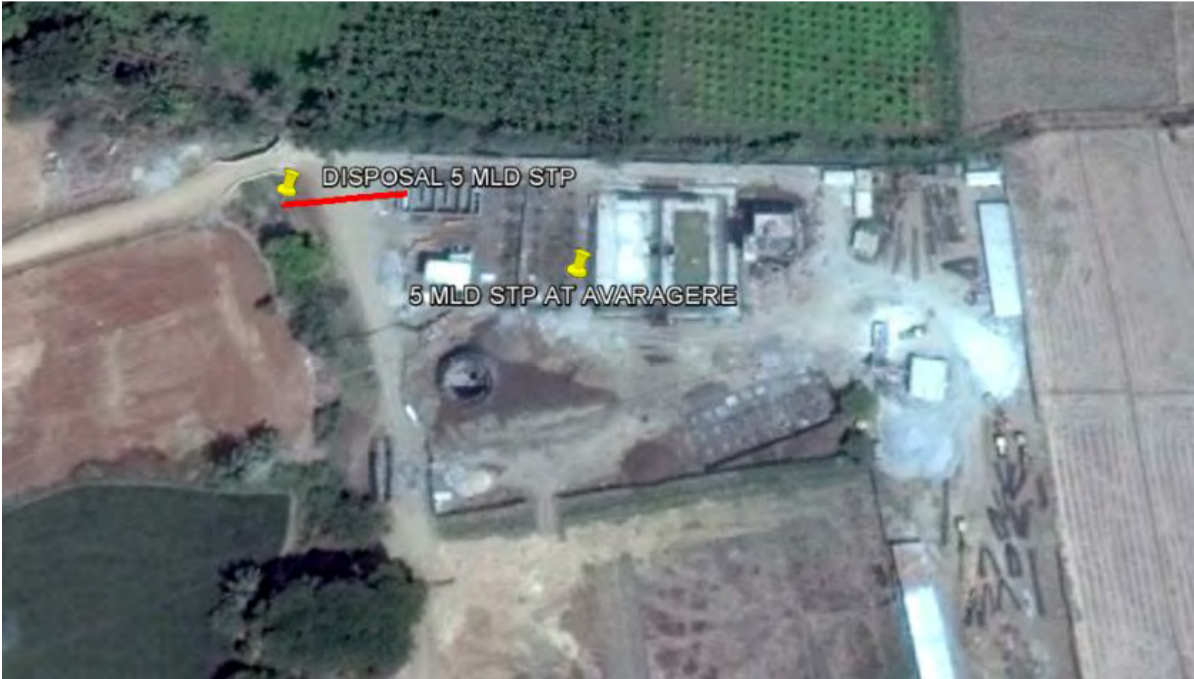
Figure 6A: Discharge point of 5 MLD STP effluent after treatment
