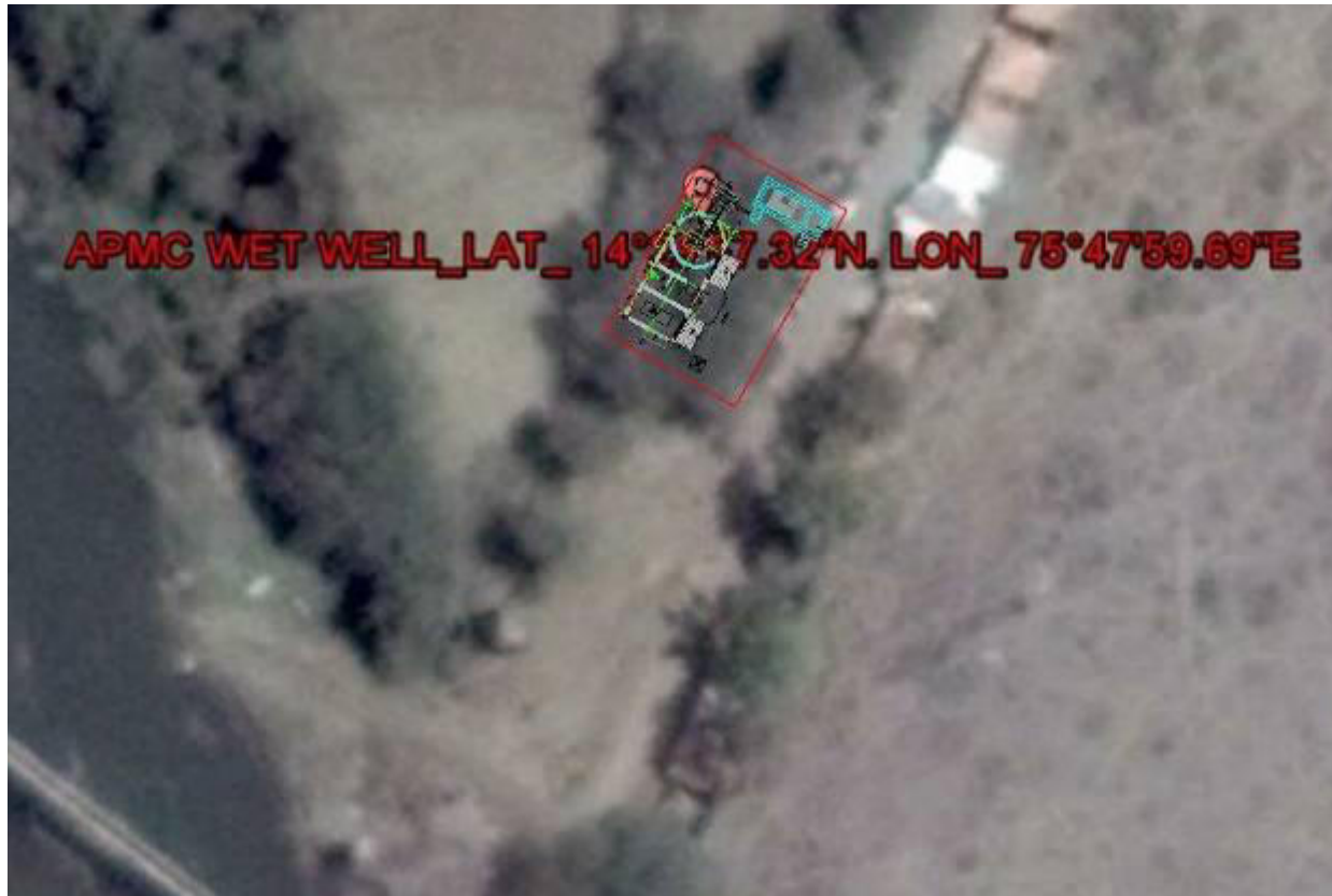
Figure 8: APMC pumping station
