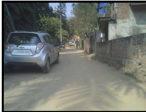
Photo 4: Water Distribution pipeline laying area at North Jyoti Nagar
