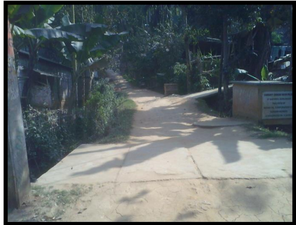
Photo 2: Water Distribution pipeline laying area at Gopalnagar
