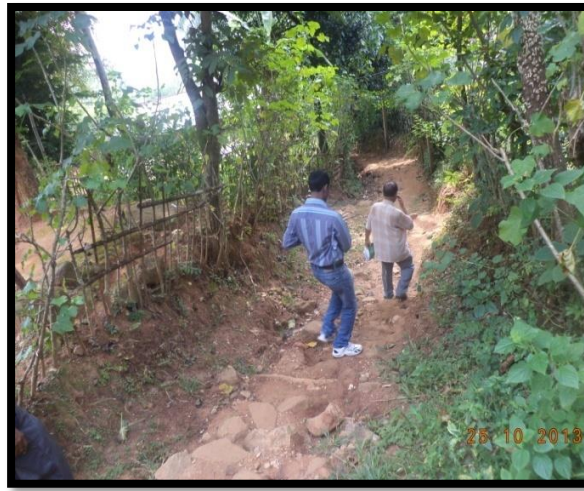
Photo 6: Water Distribution pipeline laying area at Kenduguri
