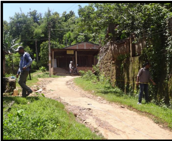
Photo 5: Water Distribution pipeline laying area at Basistha
