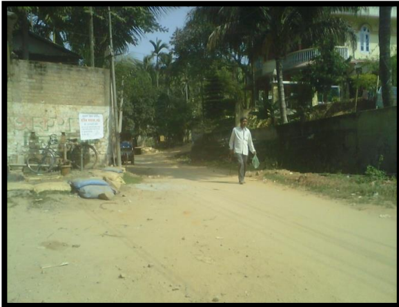
Photo 1: Water Distribution Pipeline Laying Area at Gopalnagar
