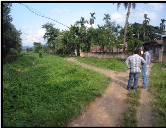
Photo 3: Water Distribution pipeline laying area at Jonaki nagar
