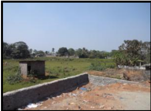
Photo 3: Proposed water treatment site at Sunshali
