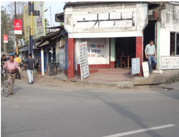
Non Existing Drain – Polo ground to 1080 chainage
