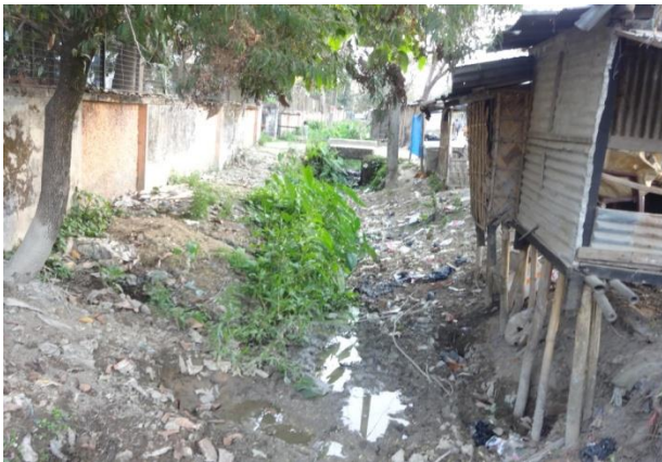
Road side vendors and status of drain at Mancota Road
