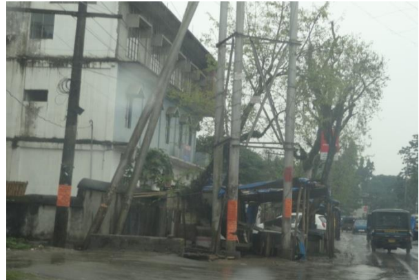
Road side vendors along the drain (Mancota Road)
