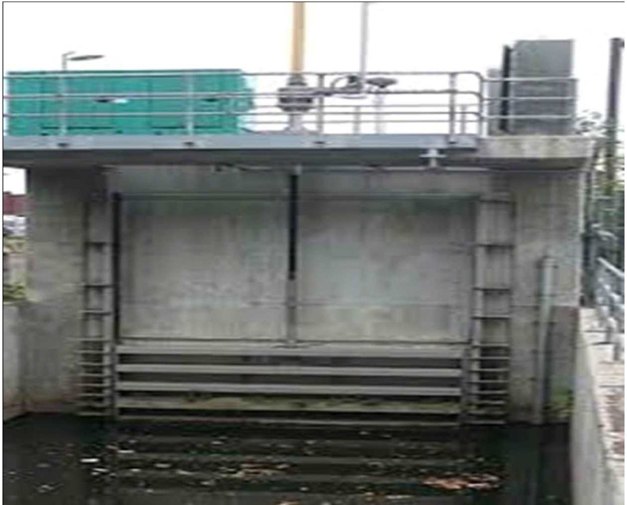
Vertical Sluice Gate Arrangement
