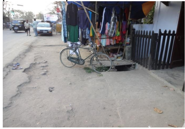
Temporary shop in the drain (AMC road)
