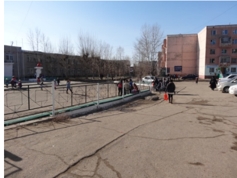
Picture 2: Iron fence, speed bump and gate to be moved
