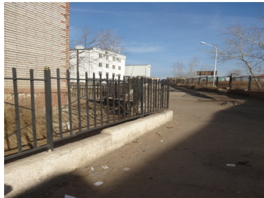
Picture 2: Iron fence and gate to be moved
