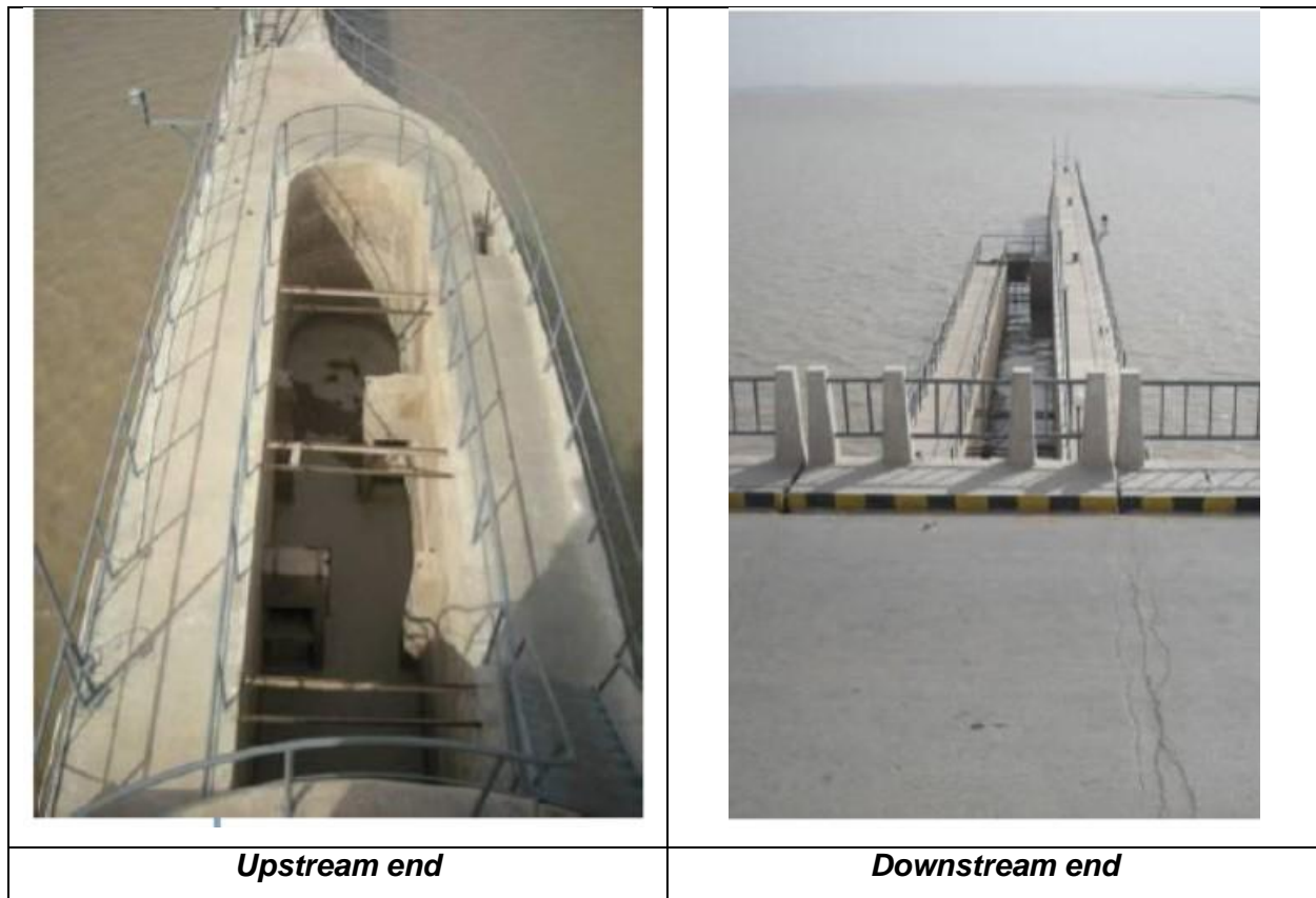
Figure 7.3: Right side fish ladder at Guddu Barrage (Gate 7)
