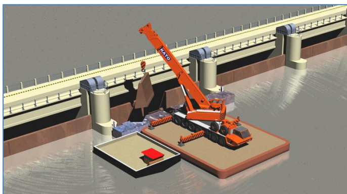
INSTALLATION OF NEW GATES
