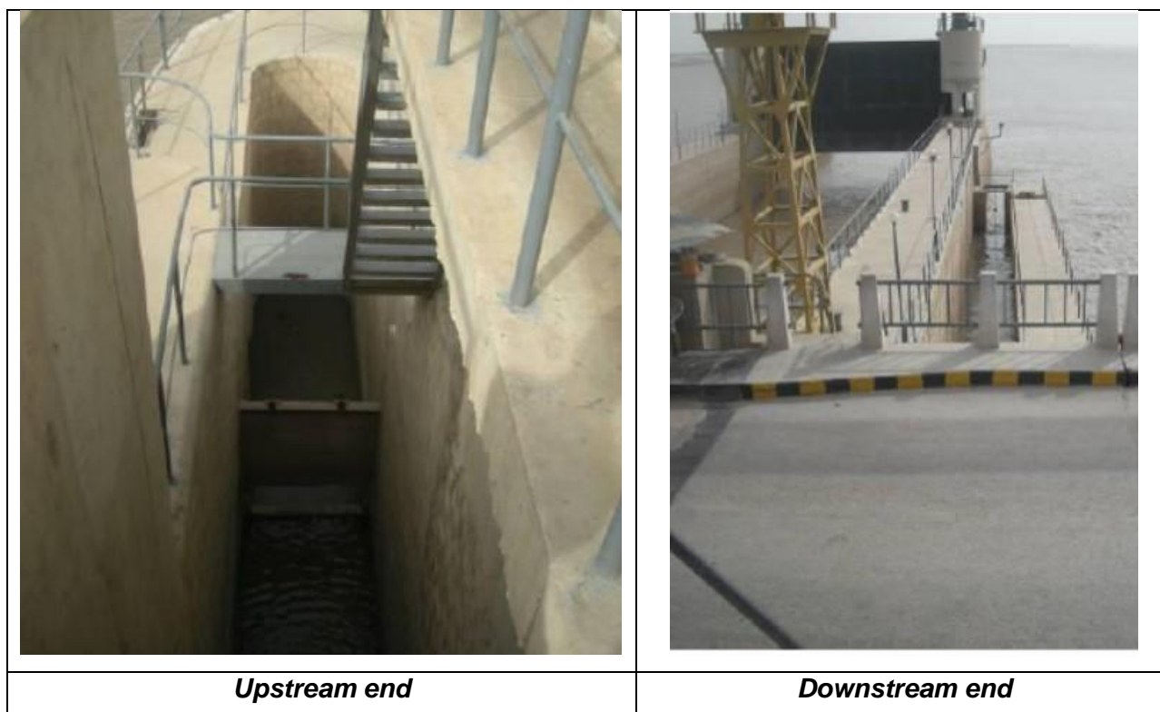
Figure 7.4: Left side fish ladder at Guddu Barrage (gate 61)
