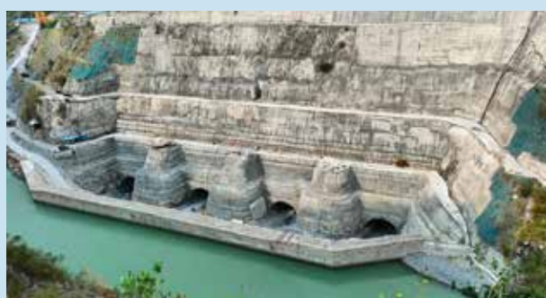
View of Concrete Lining in all limbs from the outer side of 1000 MW Tehri PSP
