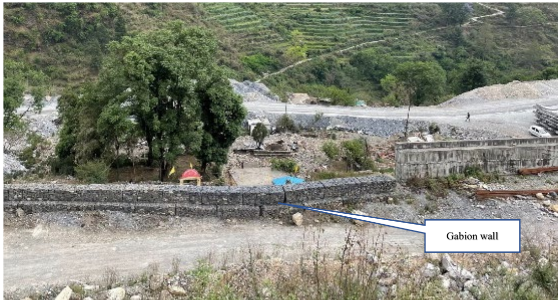
Photo 4. View of the back of the gabion wall (red roof of temple complex visible) showing that no muck is being dumped behind it
