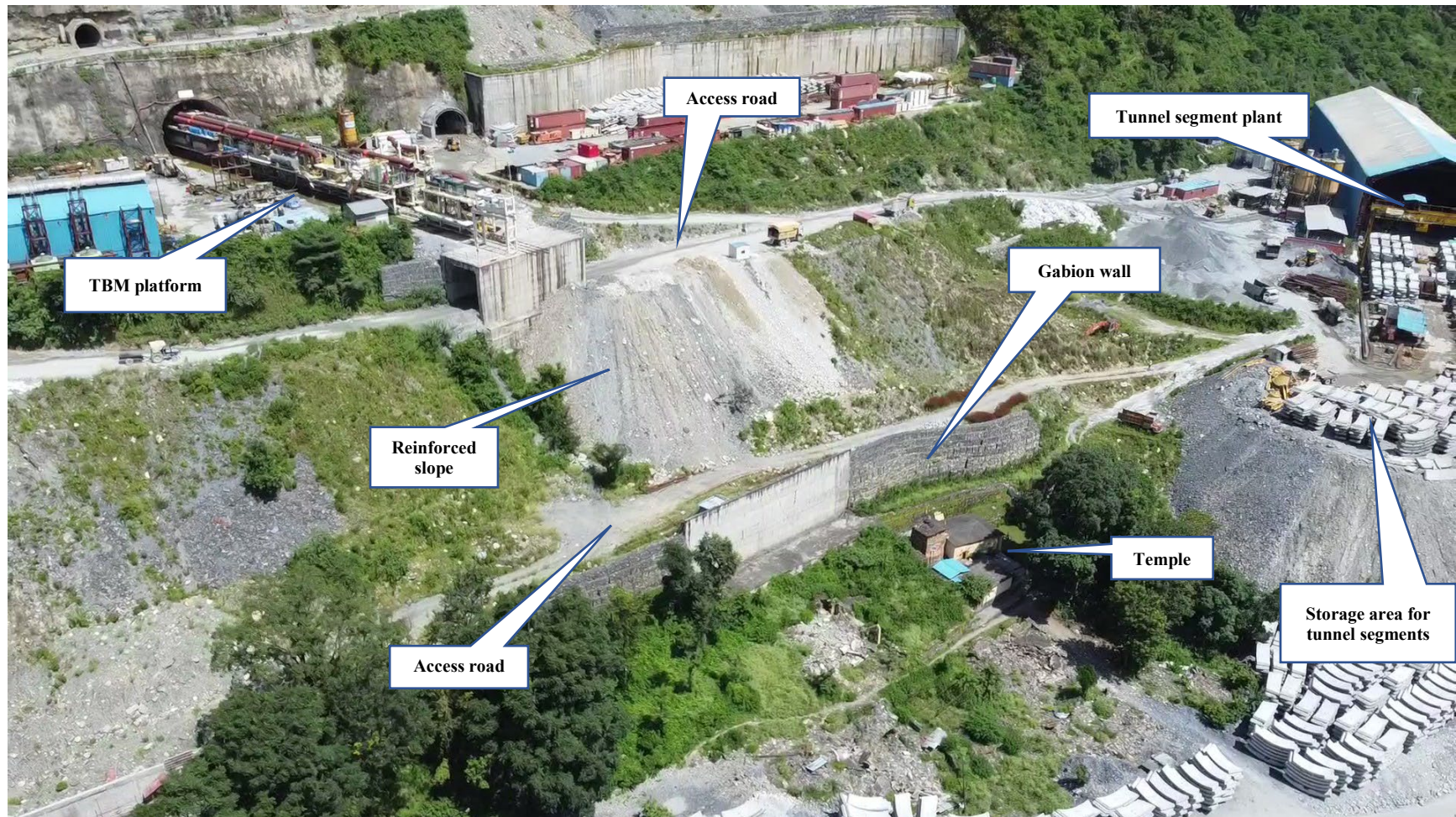
Photo 1: Aerial photo of the temple complex and the surrounding project works (August 26, 2022). No muck is being dumped behind the wall to the north of the temple complex (i.e., behind the gabion wall).
