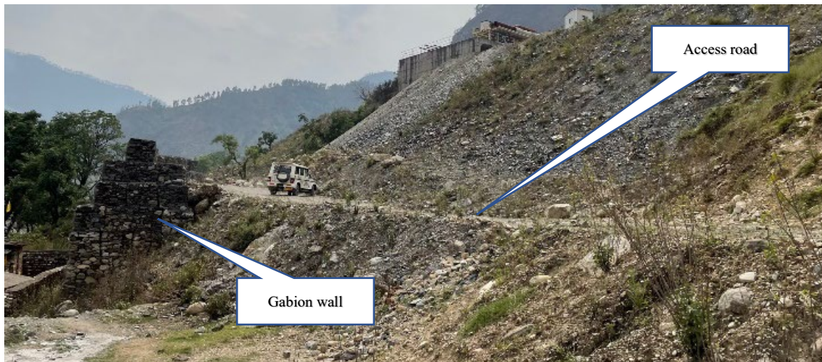
Photo 3. Cross-section view of gabion wall with access road to the right and temple complex (not visible) to the left. If the gabion wall was used to protect against stored muck, this access road would not be usable by vehicles.
