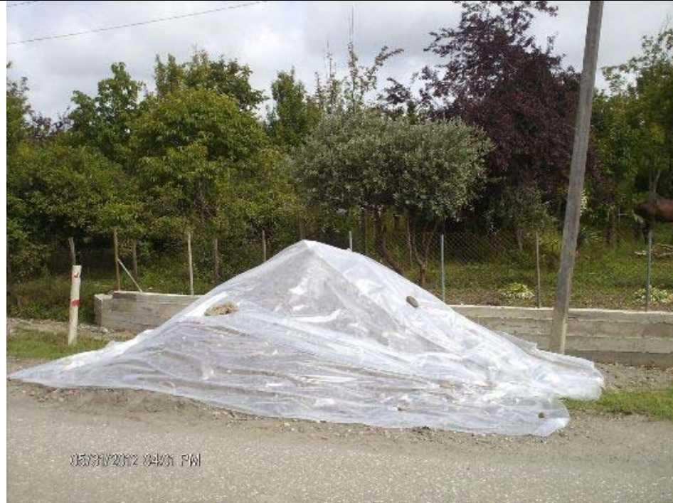
Backfilling material protected by plastic liner – protection from washout.
