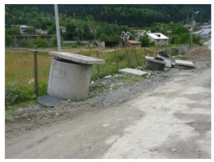
MES 02 - Improperly placed sewage system loop
