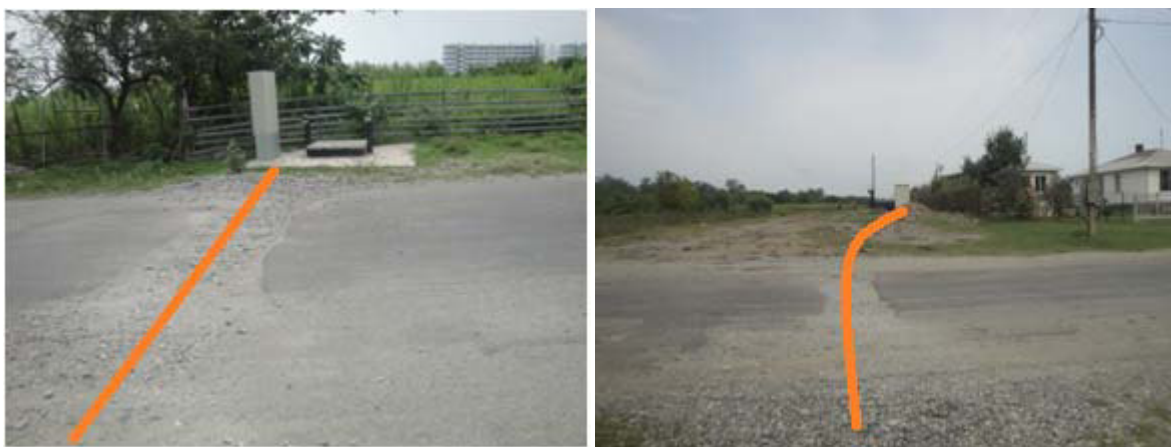
Figures 14 and 15: Degree of unsatisfactory restoration of damaged asphalt layers
