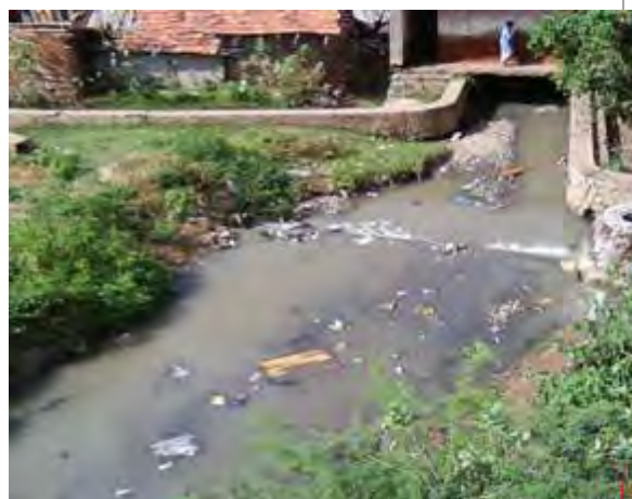
Photo 2: A view of sewage discharging to storm water drain
