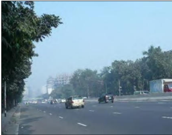
Photograph2 Km 2+000 looking north (at grade BRT 2+2)
