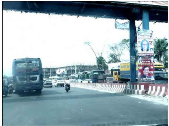
Photograph 5: Km5+200 Tongi Station Road looking north (BRT elevated 2+2)
