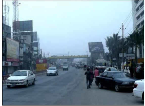
Photograph 4 Km4+300 looking south towards Tongi Bridge (eight-lane flyover at bridge, BRT elevated 2+2)
