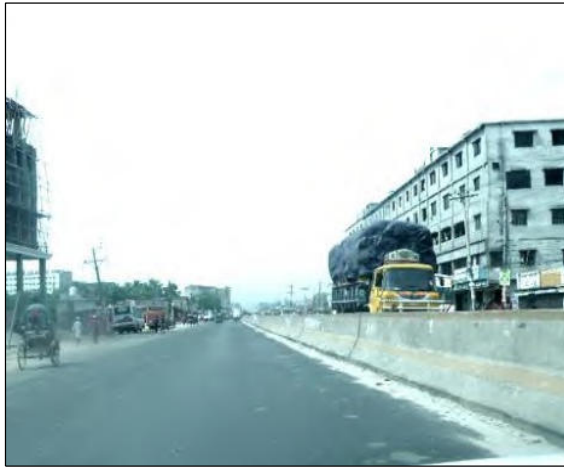
Photograph 7 Km8+600 looking north (BRT at grade 1+1)
