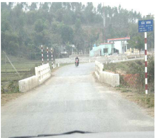
QL217 – A typical bridge
