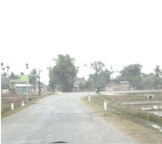
QL217 -A typical embankment
