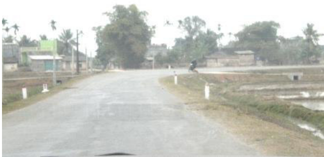
Photograph 2 QL217 -Typical embankment
