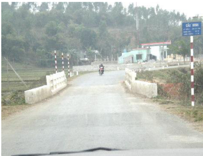
Photograph 3 QL217 -Typical bridge
