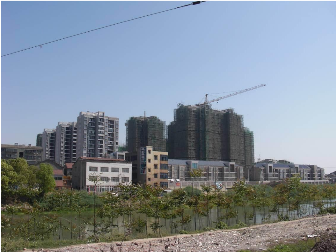
Picture 6-1 The resettlement site of Binhu community in construction
