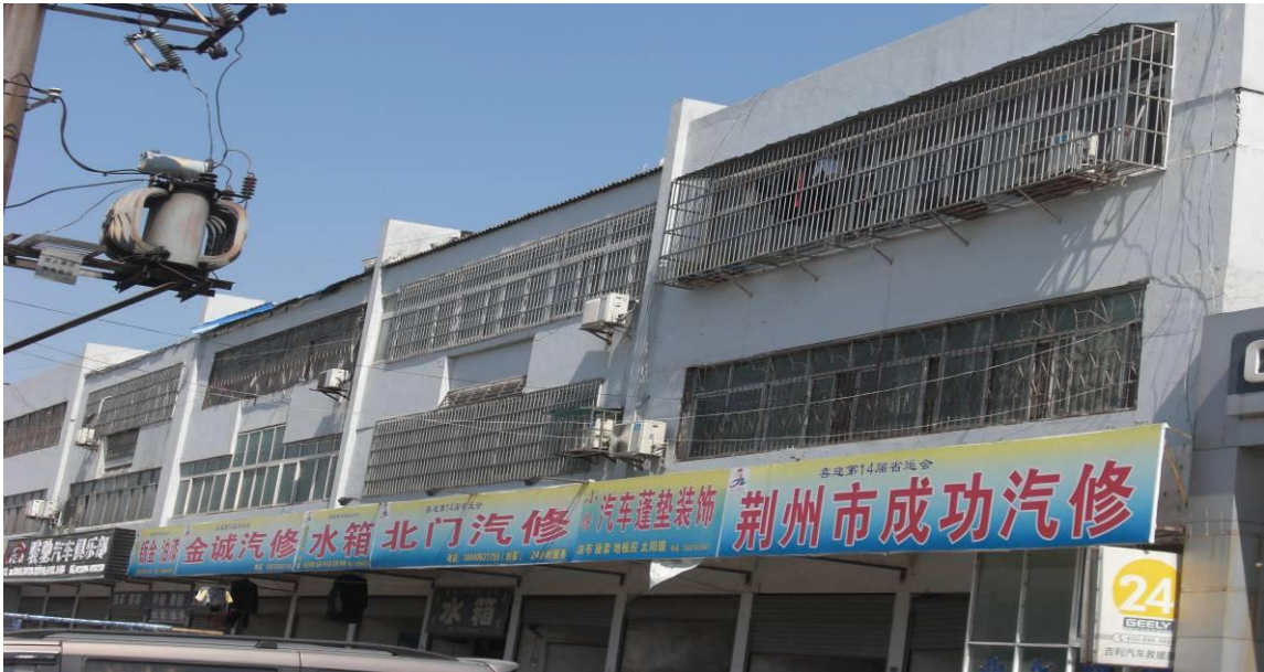
Figure 2-8 Business buildings of Four Lakes Administration required to be demolished
