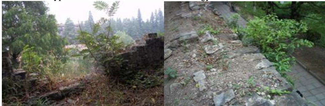
Current conditions of pinion wall and abutment wall
