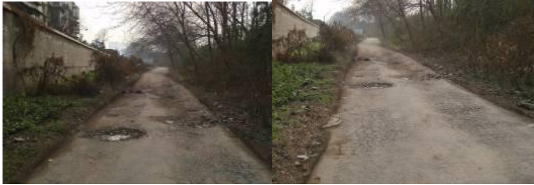
Dirt road section of the Inner Ring Road
