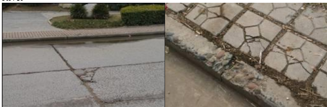
Current conditions of the surface of Inner Ring Road
