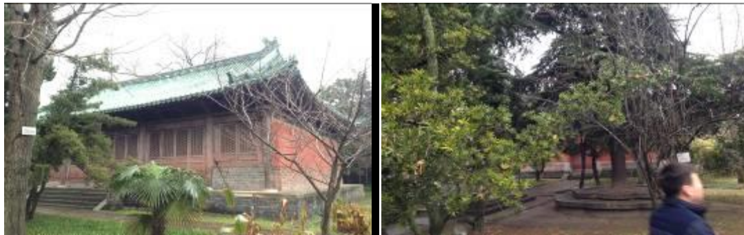
Figure 3.7-7 Current conditions of Kaiyuan Taoist Temple
