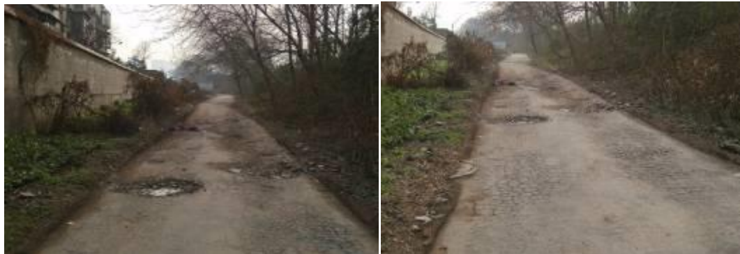
Figure 3.7-13 Dirt road section of the Inner Ring Road
