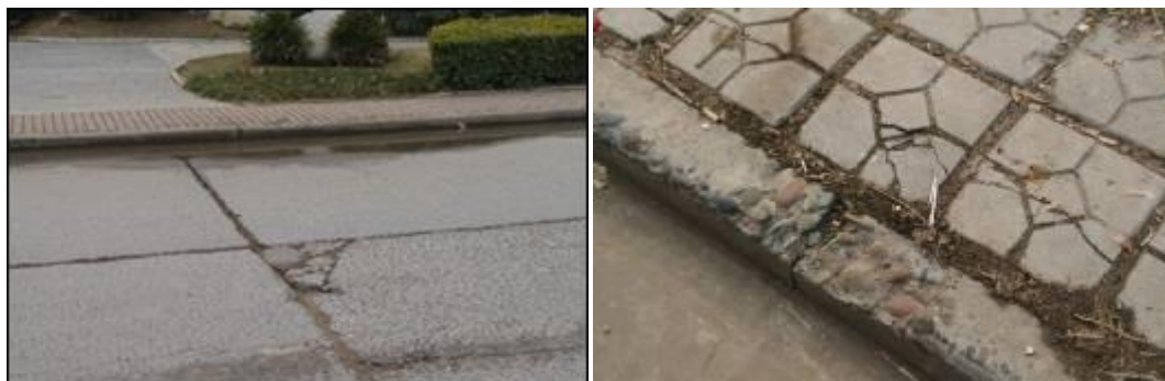
Figure 3.7-12 Current conditions of the surface of Inner Ring Road
