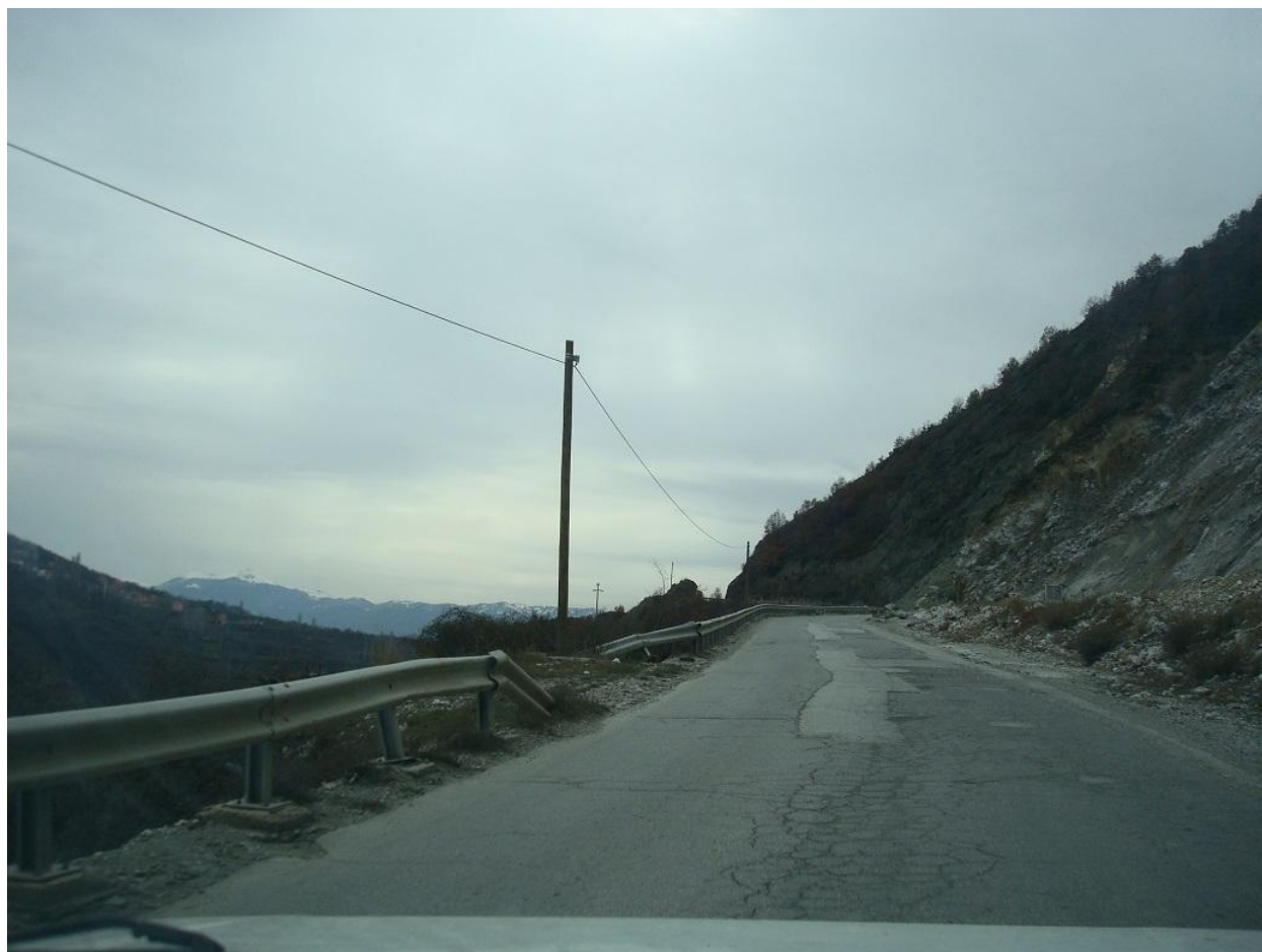
Figure 5 Current state of the road section Boskov Most - Debar
