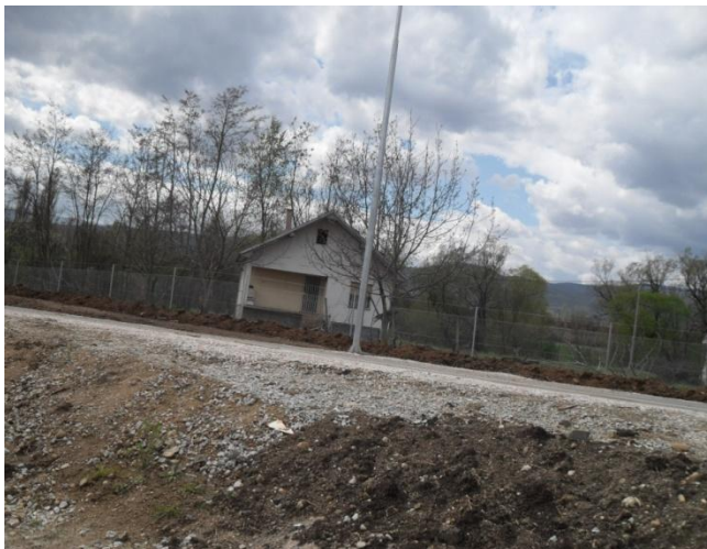
Figure 3 Part of the station km 1+280 to km 1+370
