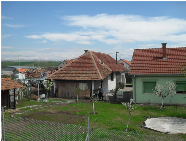
Figure 6 Part of the station km 7+348 to km 7+525
