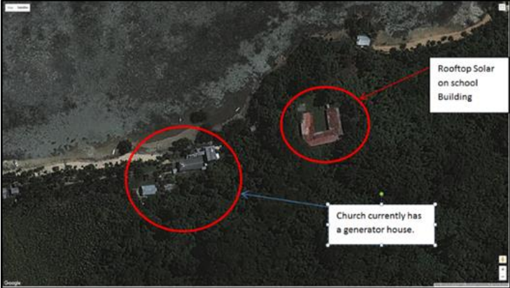
Figure 16. Aerial photo of Walung school and church. The solar PV installation will be on the roof of the school.
