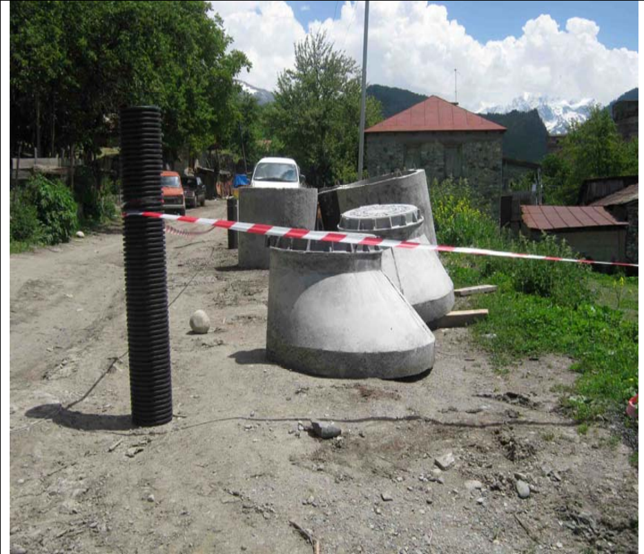
A view of material stocking area.
