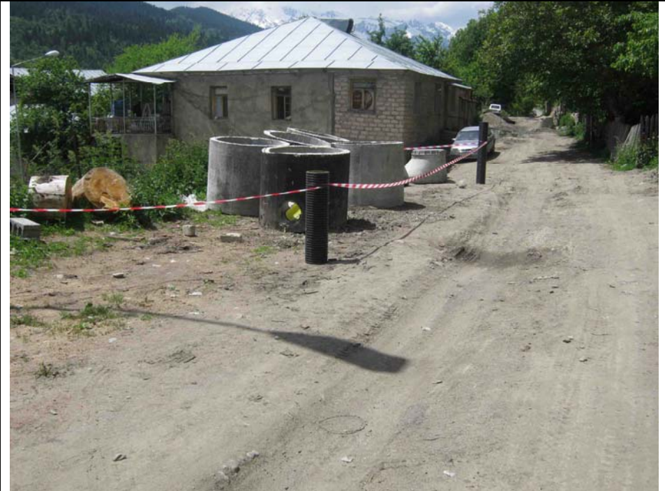
A view of material stocking area.
