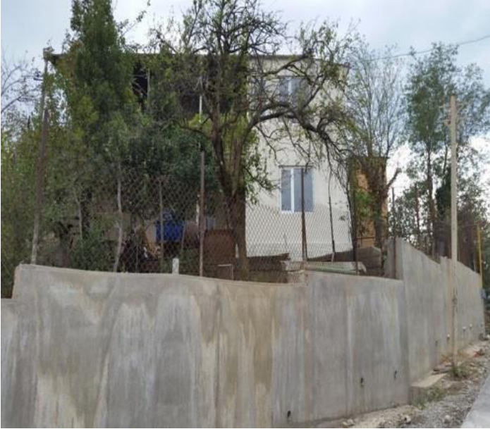
Kutaisi Reg-01: Rehabilitated house and wall of #9a Koguashvili street
