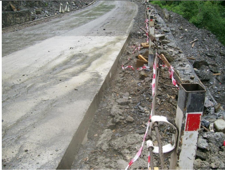
Rectification of concrete pavement
