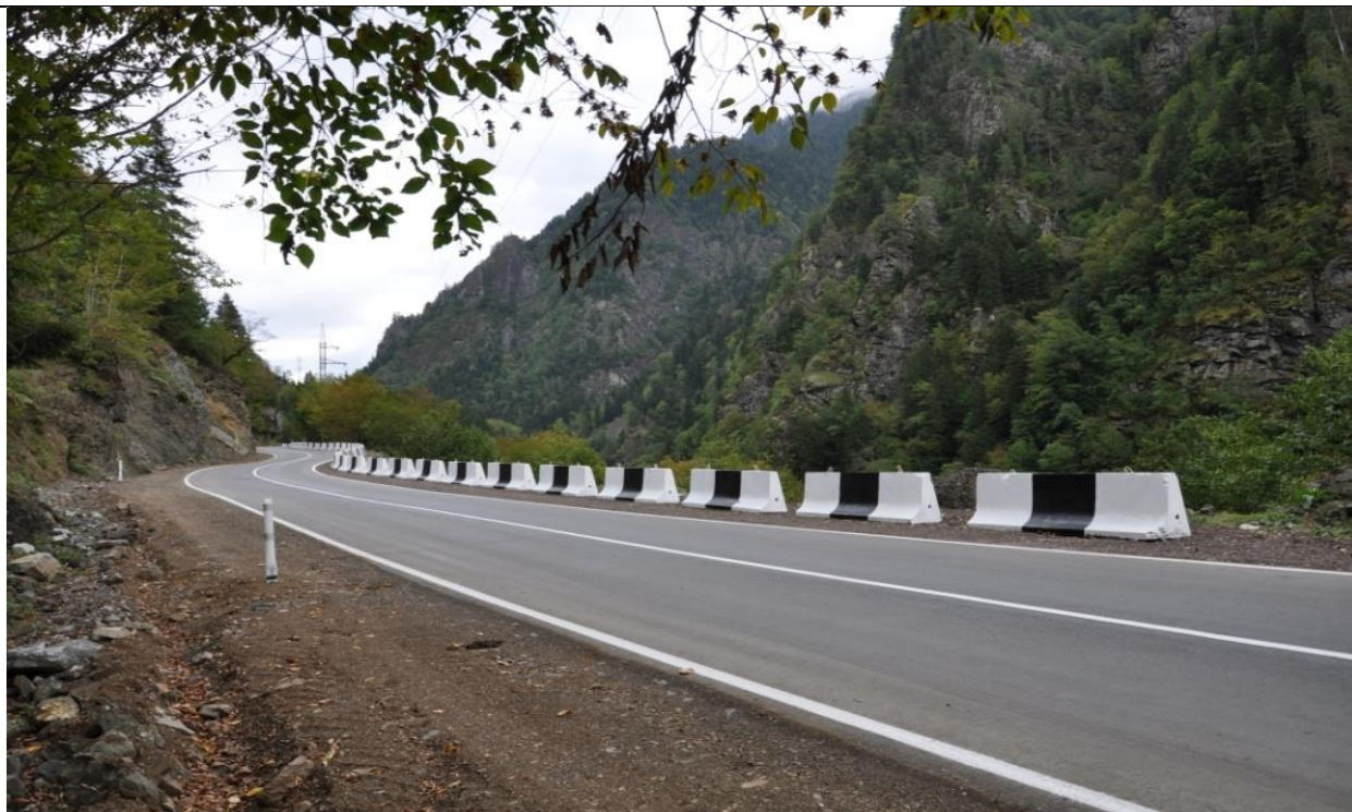
Completed section of Lot 1
