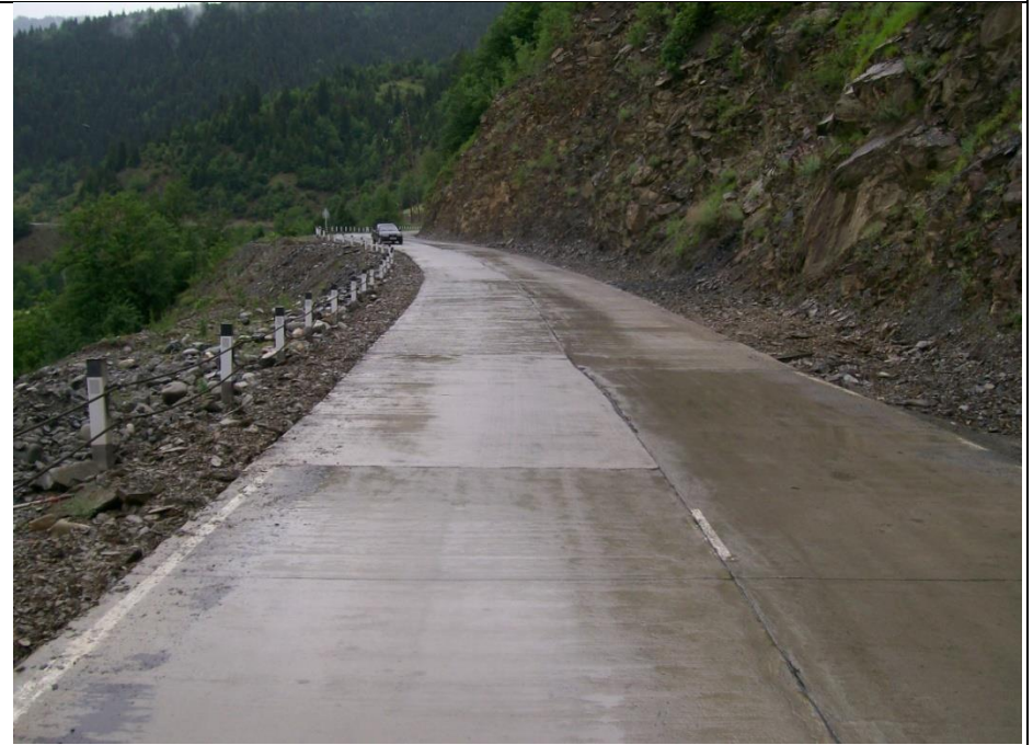
Remedial pavement works
