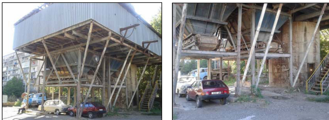
Figure 24.- Shaft n° 51. Construction site
