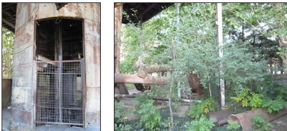
Figure 23.- Shaft n° 50. Construction site
