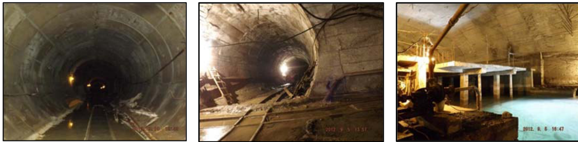
Figure 37.- Water in the tunnel and University Station
