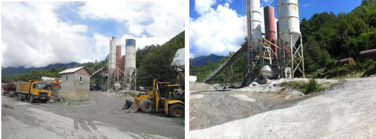
Fig. 27 and 28. Operating building camp of ENGURI 2006 LTD. and related infrastructure
