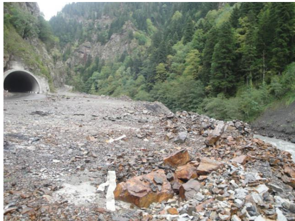
Fig. 6. KP 89 entrance to the tunnel from Khaishi side
