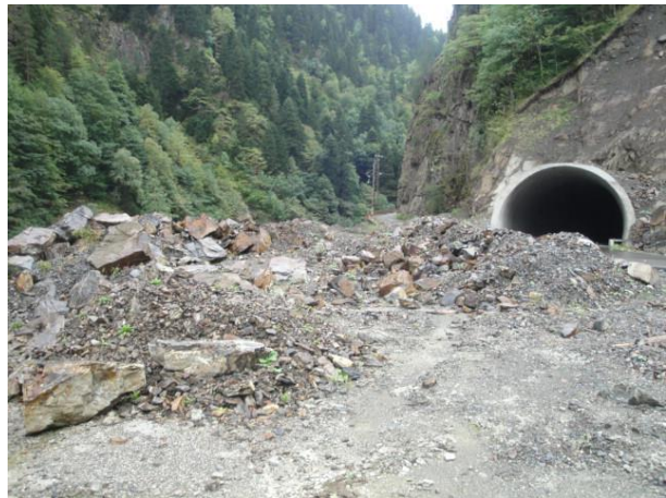
Fig. 4. KP 89 Entrance to the tunnel from Mestia side
