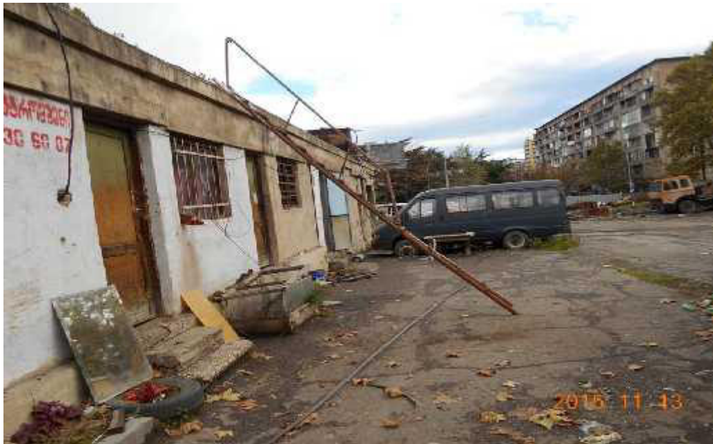
Photograph 1. Area close to the offices that must be cleaned. Details of abandoned vehicles
