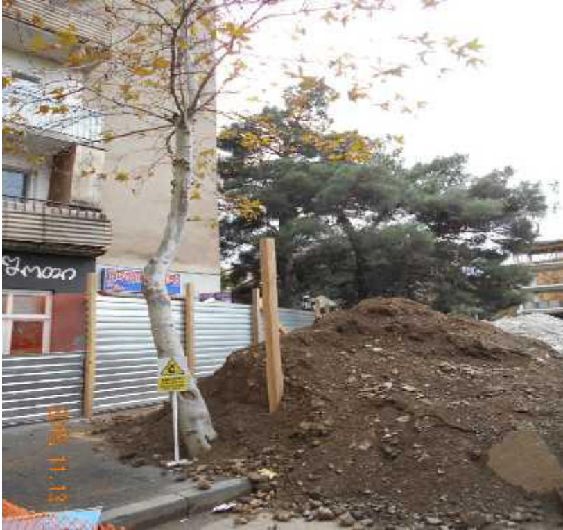
Photograph 7. Three that is going to be affected by the works and shall be cut later on
