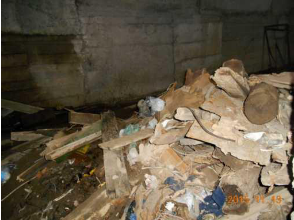
Photograph 5: area behind one of the air conduct. There is accumulation of wastes that must be removed.
