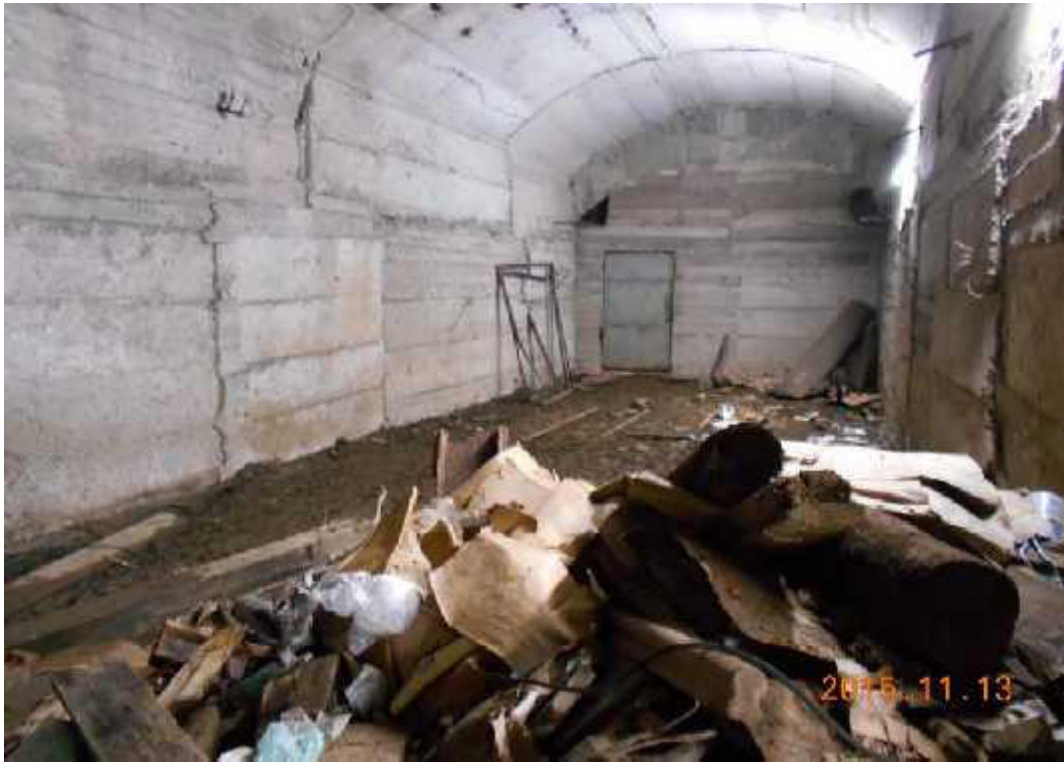
Photograph 9: Area inside the tunnels with rubbish accumulation that must be removed
