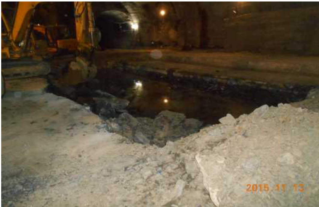
Photograph 4: Area inside the tunnels with zones of water accumulation
