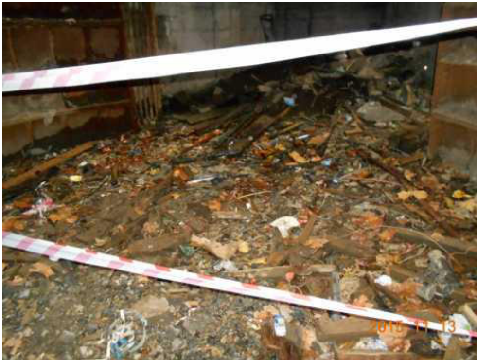
Photograph 6: Details of the area mentioned in the photograph 5.
