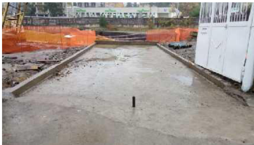
Picture 1: Vehicle washing area
