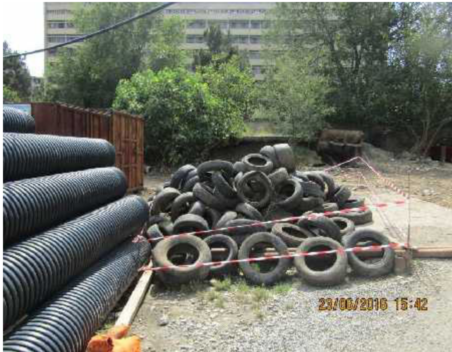
Photograph 4. Wheels disposal waiting to be removed
