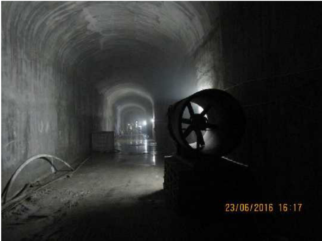
Photograph 5. Fans off when the tunnel is dusty
