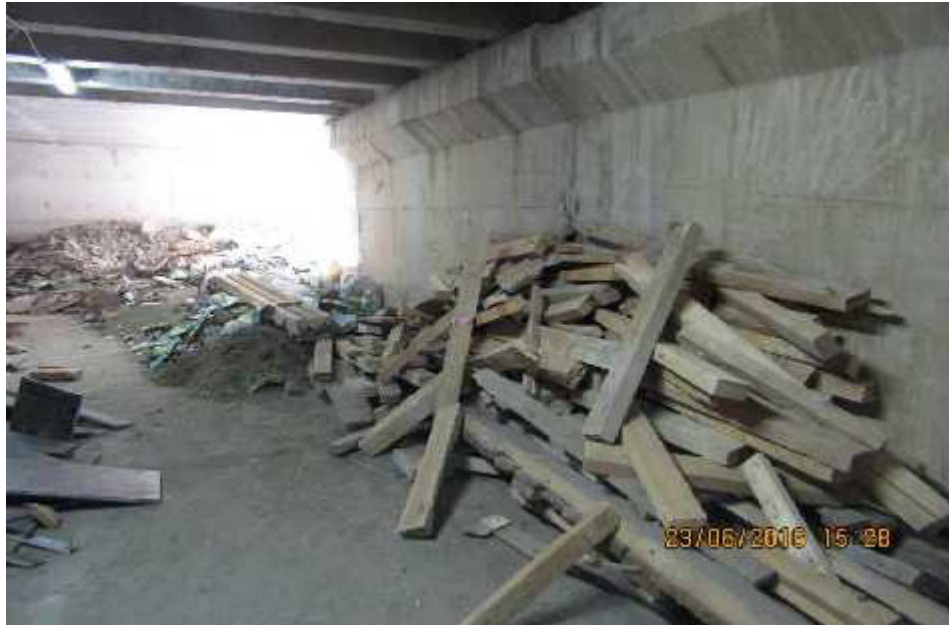
Photograph 3. Waste disposal inside the tunnel
