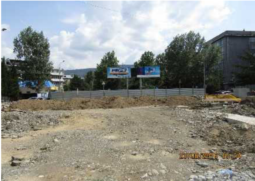
Photograph 1: Working area in good state
