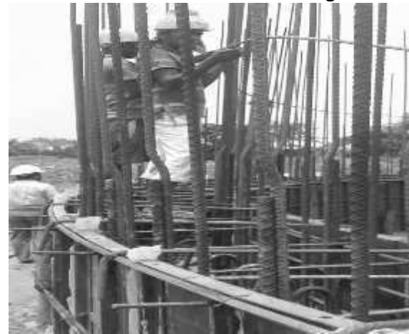
Use of PPE by worker at pumping station construction site
