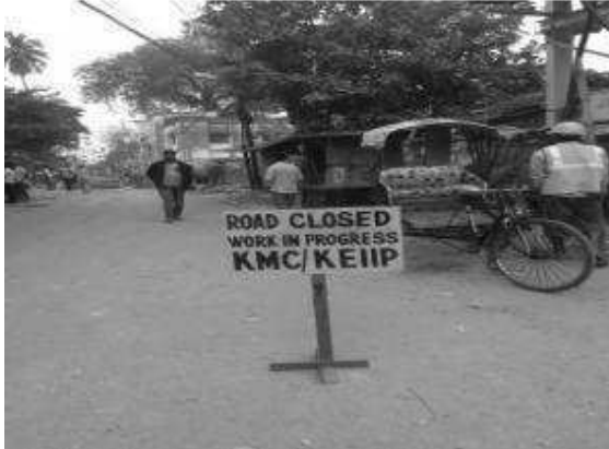
Caution board noted at working area
