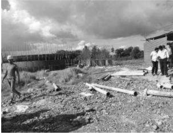
Improvement of housekeeping is required within labour camp
