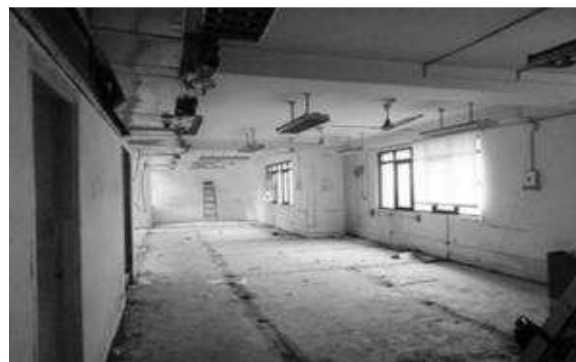
Work continued renovation of KEIP office
