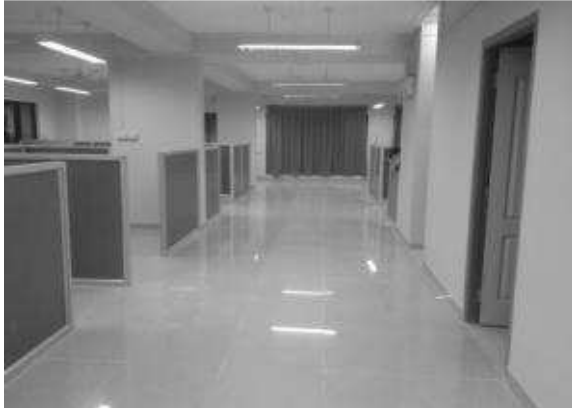
Finished floor before handed over
