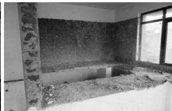
Work continued renovation of KEIP office. Generation of dust noted
