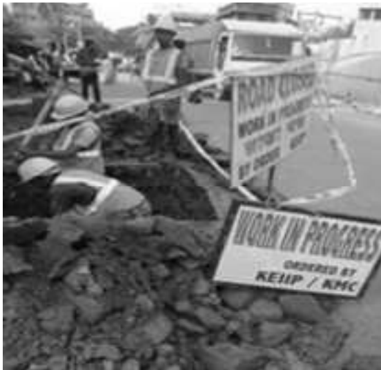
Work in progress at Gardenreach area for GAP sewerline. Use of PPE, caution board and tape noted
