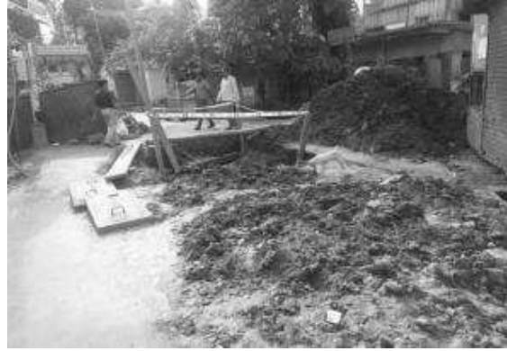
Partial road closure noted. Use of caution tape noted. Excess earth needs to be removed from construction site
