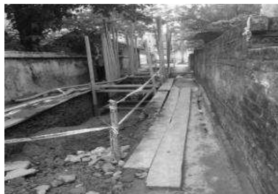
Access available at working site
