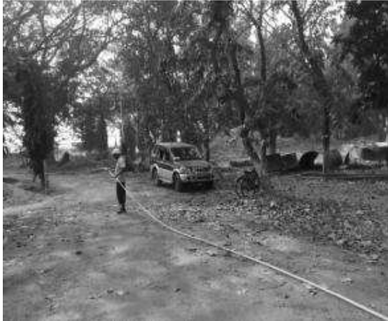
Water sprinkling at road construction site for suppression of dust
