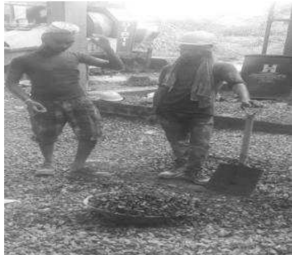
Use of PPE by workers
