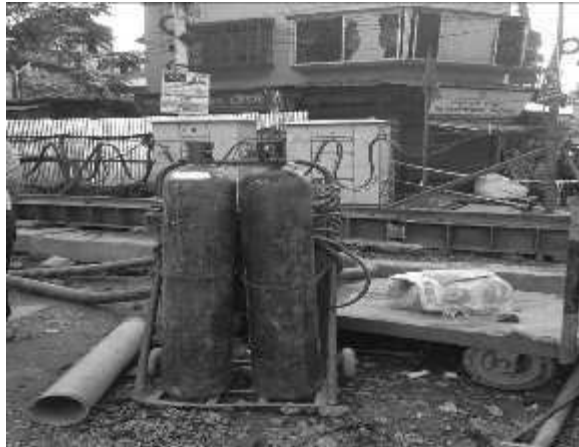
Proper storage of cylinder noted at shaft 9 Buro Ashwattala of DH Road micro tunnelling location
