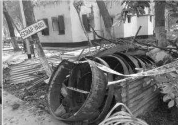
Separate storage of scrap materials at working site
