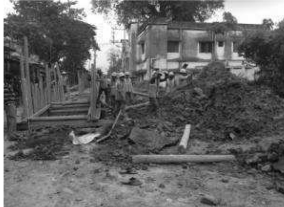
Use of PPE by workers at site
