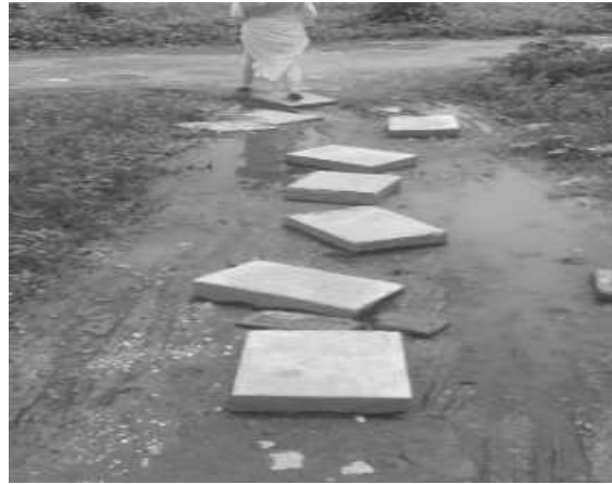
Temporary access provided during rains
