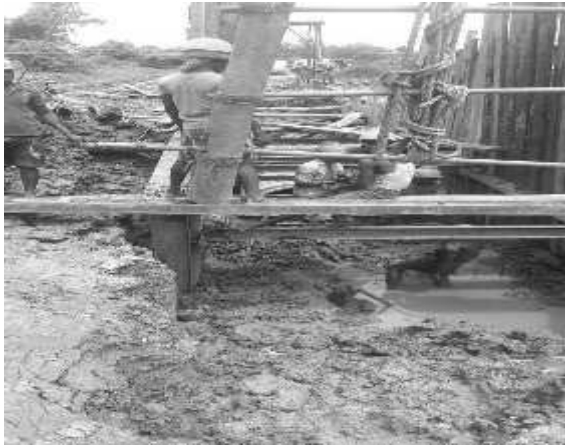
Pipe laying work within treatment plant area. Partial use of PPE noted. Proper dress need to be maintained
