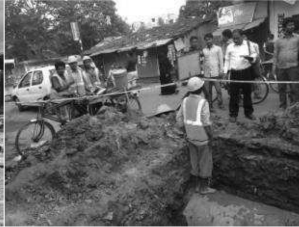
Caution tape and use of PPE by workers – noted at pipe laying area
