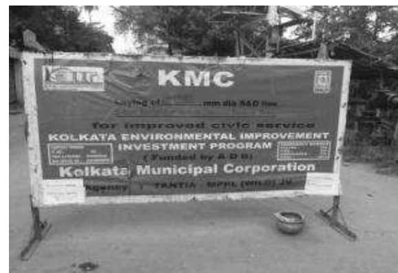
Display board noted at pipe laying area
