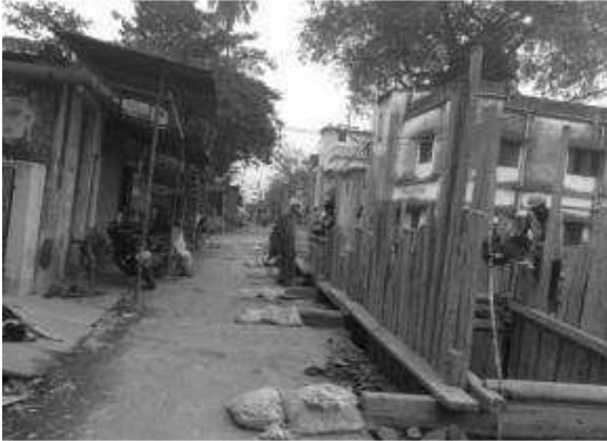
Access available at working site
