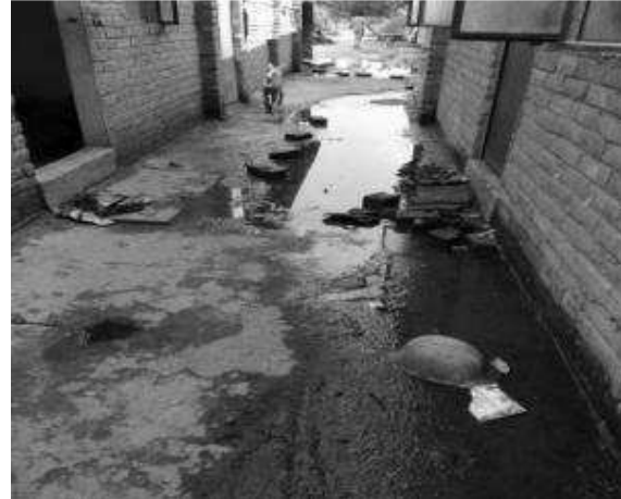
Water stagnation within the labour camp – needs discharge
