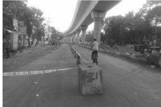
Road divider used with proper colour code at DH road working site
