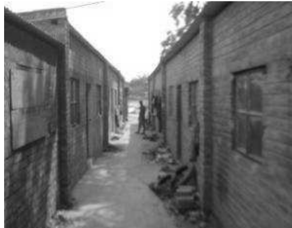
Labour camp – some improvement of housekeeping should be required
