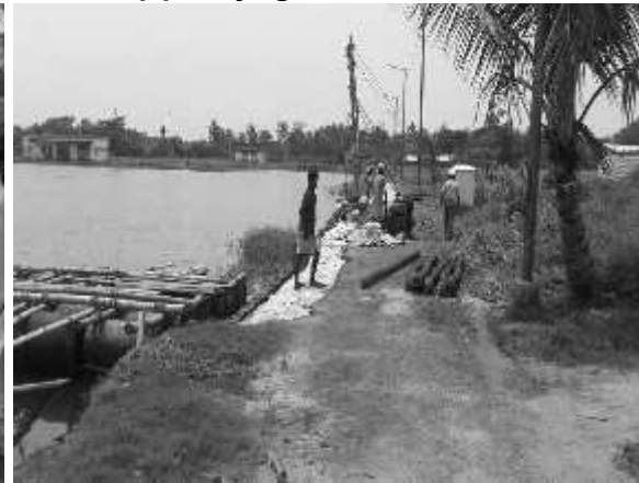
Access road maintained at working area
