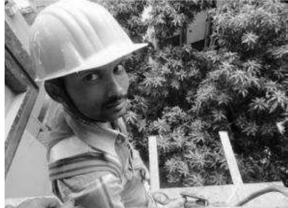
Use of PPE and safety belt by workers during outside work
