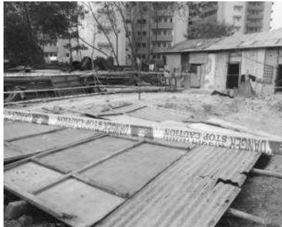
Use of caution tape and demarcation of camp at Joka Ps area
