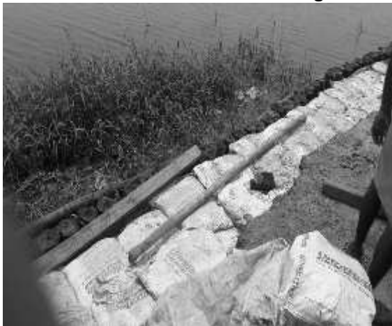
Stabilization work done near STP location of Keorapukur
