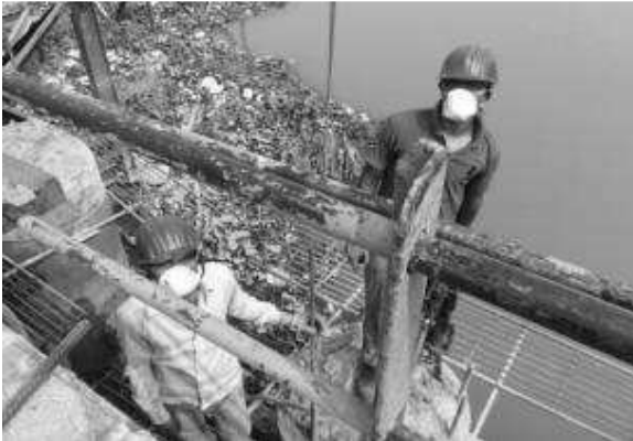
Use of PPE by worker during work at jetty area
