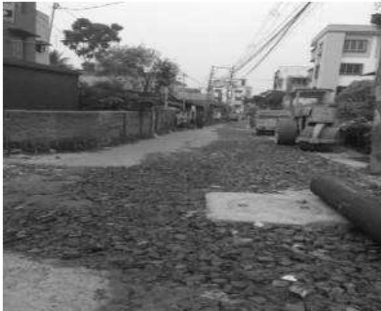
Road restoration done. Removal of excess earth from road - noted
