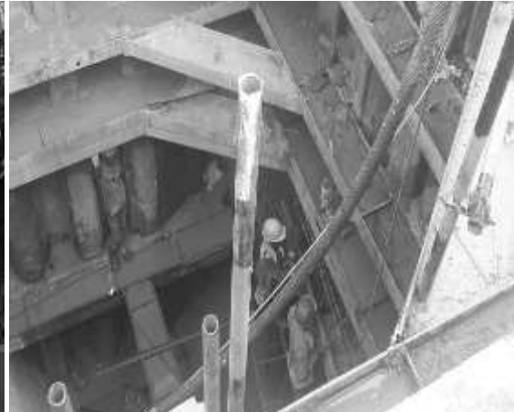
Worker with proper PPE engaged in welding at Shaft 8 of DH Road
