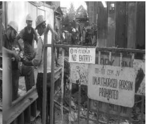
Placement of proper display board with complete road closure at Shaft no 9
