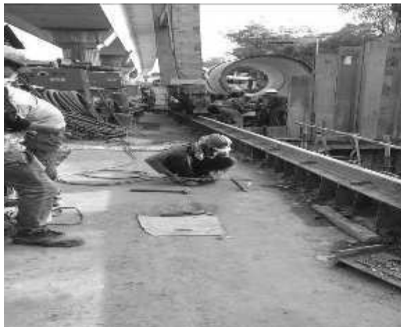
Worker with proper PPE engaged in welding at Shaft no. 8, Buro Ashwattala
