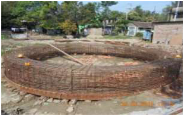
Reinforcement binding in curb in JackPush (Garden Reach)
