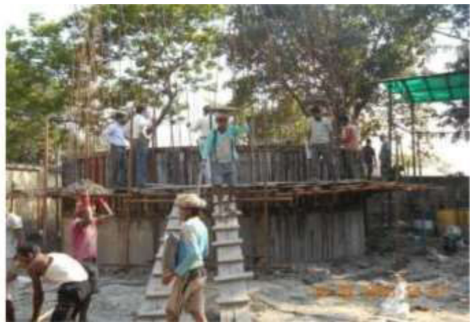
Concreting of R.P. Wall (Santoshpur)
