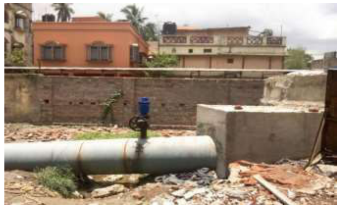
Sewage main at Santoshpur P.S
