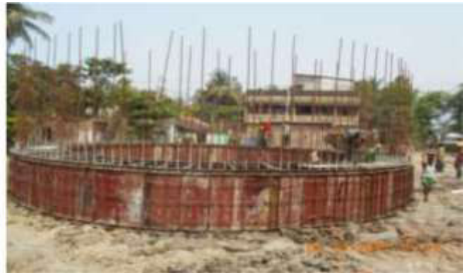
First lift of JackPush Wall (Garden Reach)
