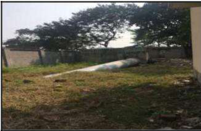
Final Micro-tunneling pipeline
