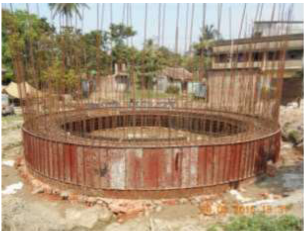
Shuttering of curb in JackPush (Garden Reach)
