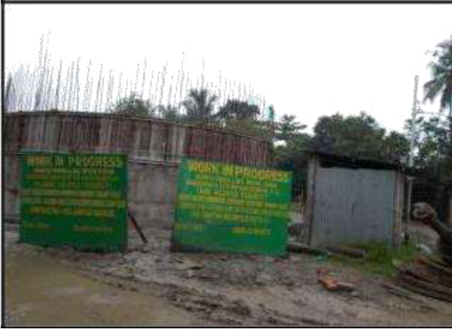
Work in Progress in Garden Reach
