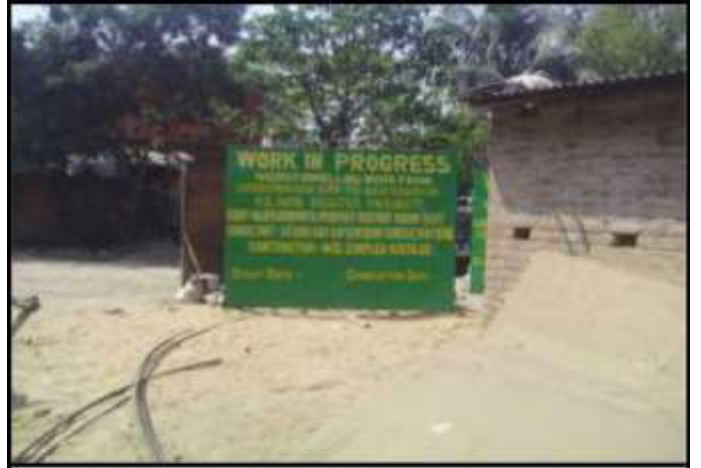
Work in Progress in Santoshpur
