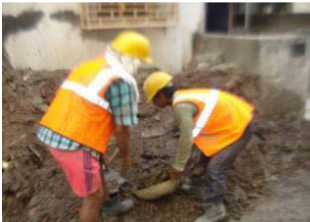
Partial use of PPE by worker
