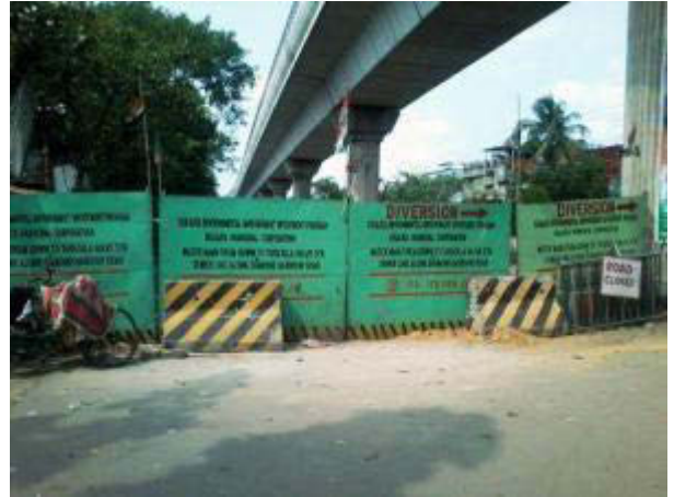
DH road shaft no 9- barricade with work detail display
