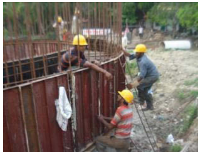
Use of PPE by worker noted
