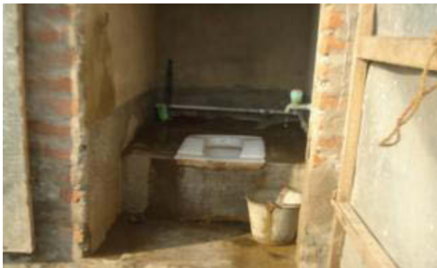
Toilet facility for worker
