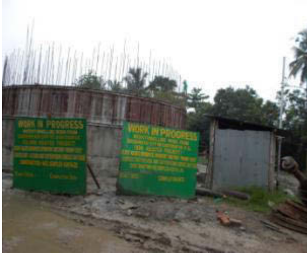
Work display board at working site
