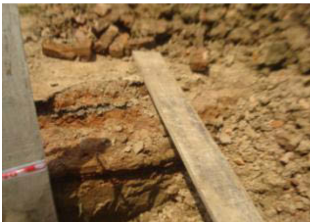
Temporary wooden platform provided for crossing over excavated area
