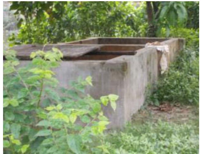
Water storage tank at labour camp
