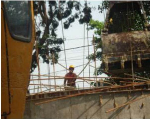
Partial use of PPE
