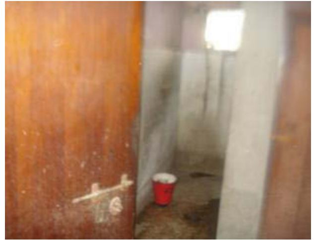
Available toilet used by Labourer
