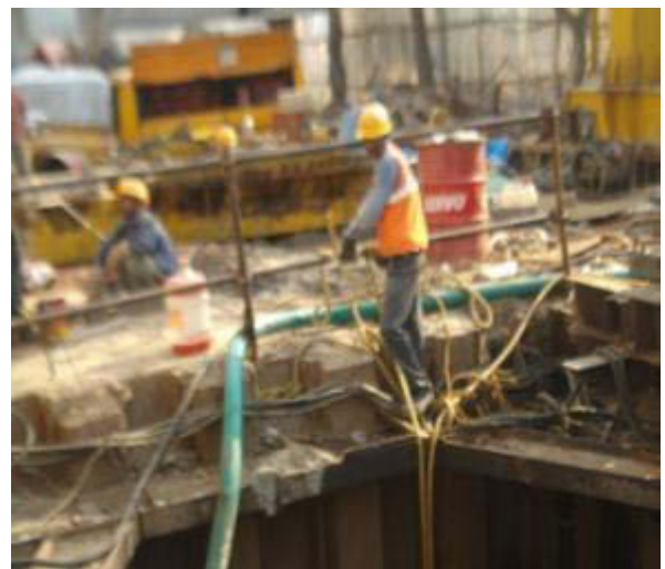
Use of PPE by workers noted
