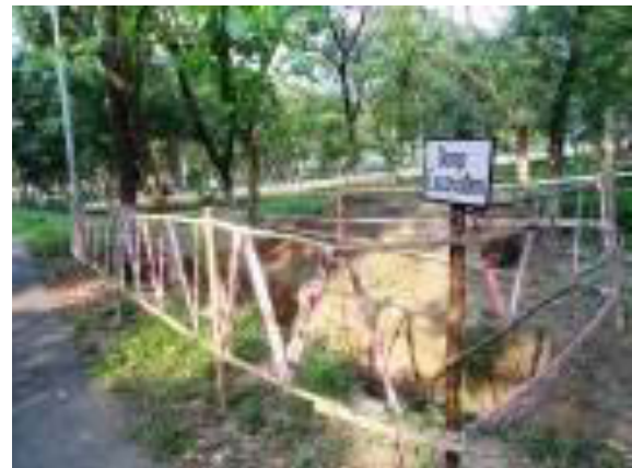
Barricading around Trial Pit
