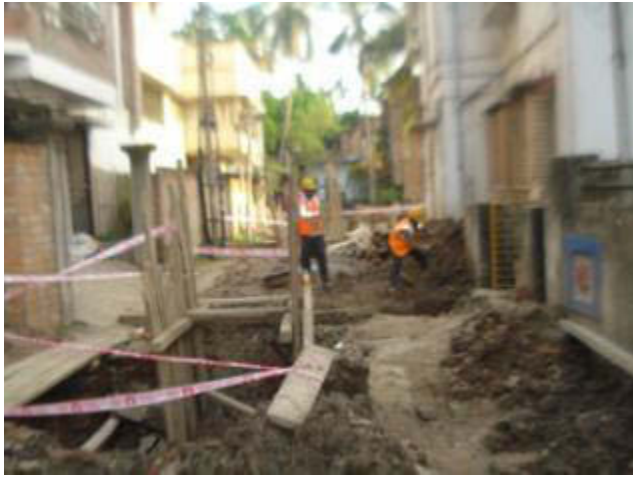
Use of PPE and temporary caution tape
