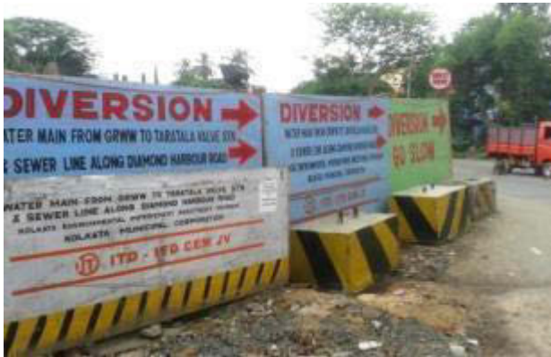
Taratala Road shaft 9 – Diversion board with hard barricade
