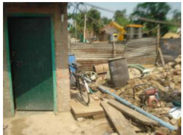
Improvement of housekeeping is required
