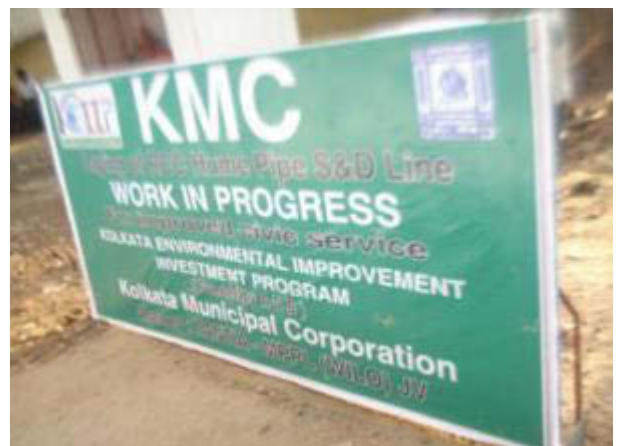
Road closure by work display board
