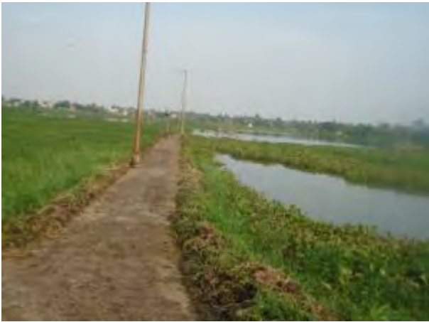
STP Ponds with full of sludge and water hyacinth
