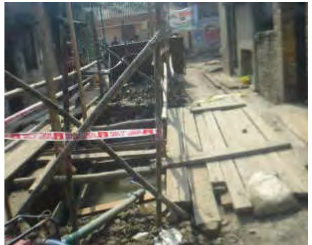
Hard barricading and wooden platform for access to site- noted
