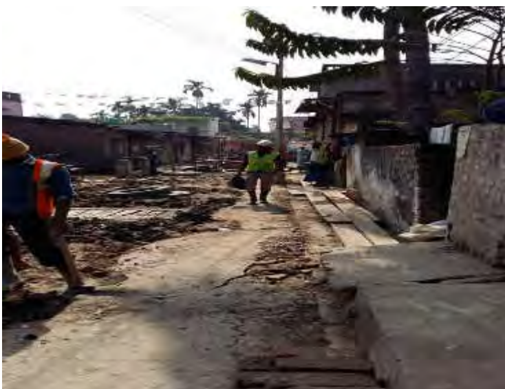
Drains are covered with wooden plate at working site after necessary instruction
