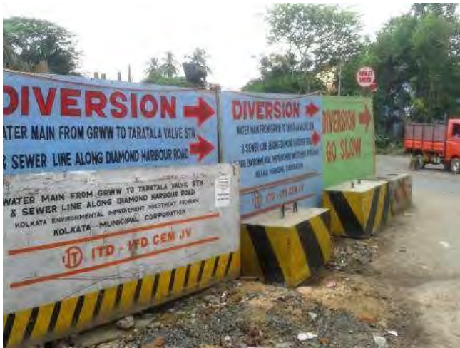
Hard Barricading with diversion sign at Taratala Road
