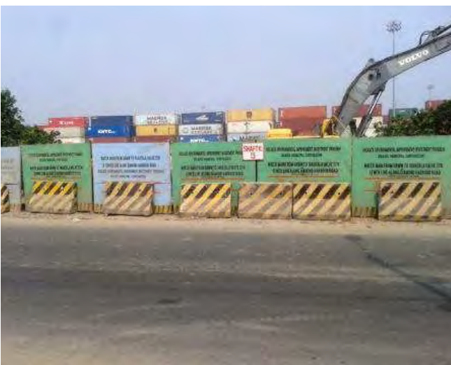
Hard Barricading Taratala Road shaft 5
