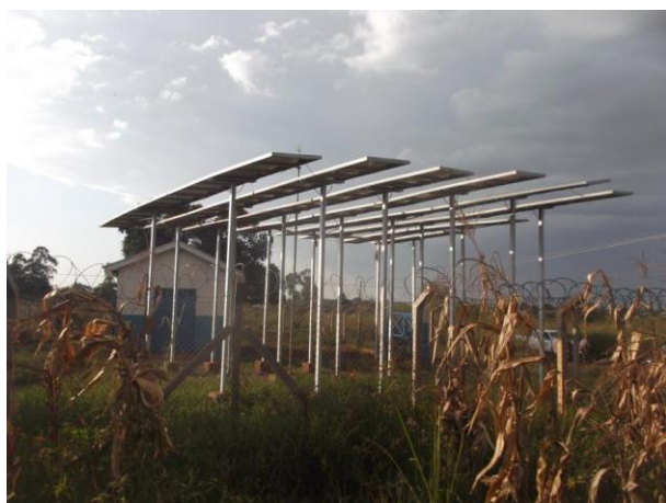
Figure 8: Water pump in Kiryandongo Refugee Settlement powered by Solar Energy
