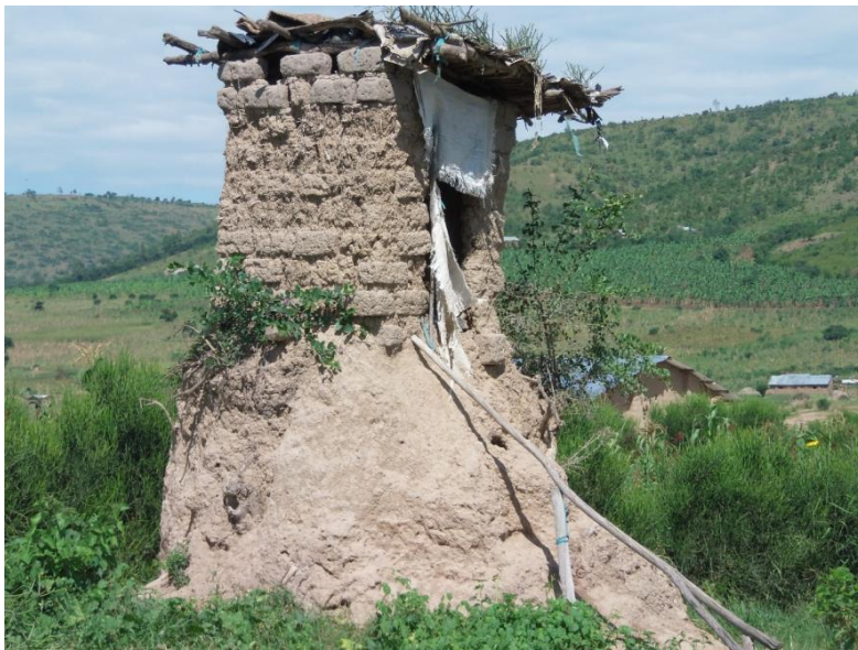
Figure 4: A typical latrine built on an anthill
