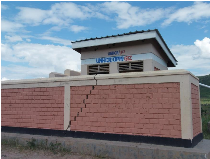
Figure 3: One of the latrines with a damaged superstructure
