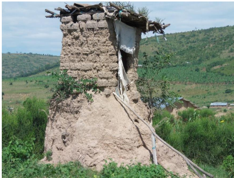
Figure 23: A typical latrine built on an anthill
