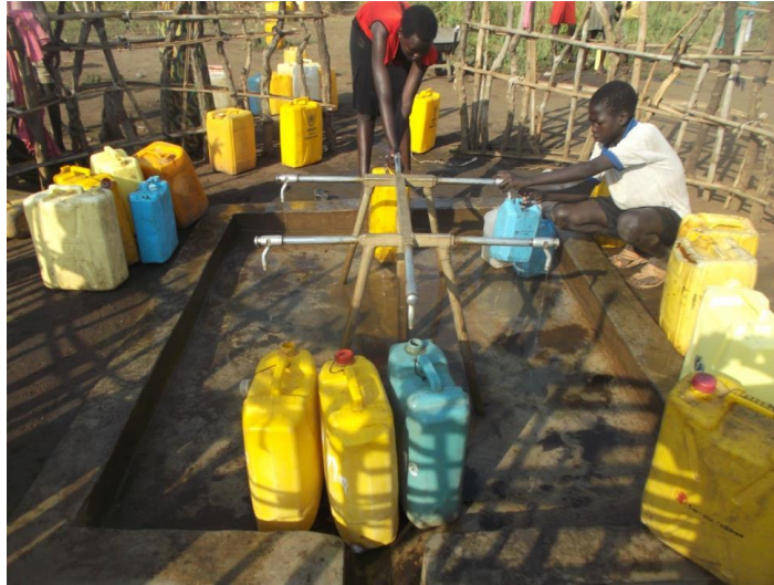
Figure 5: Water point in Nyumanzi refugee in Adjugopi Parish, Dzaipi Sub-county, Adjumani District
