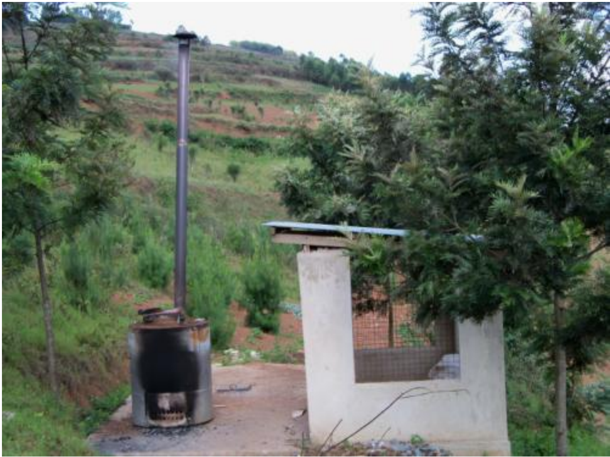
Figure 39: MAK IV Incinerator
