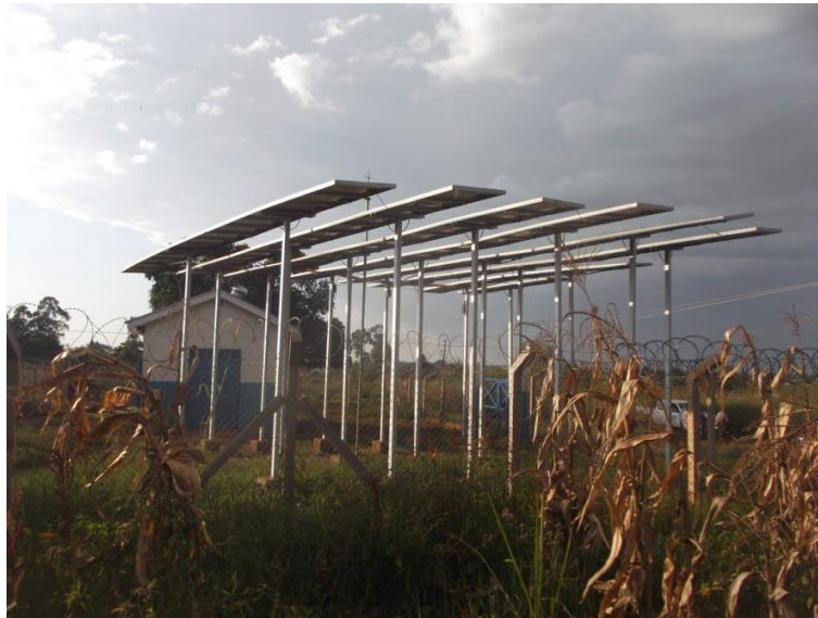
Figure 15: Water pump in Kiryandongo Refugee Settlement powered by Solar Energy
