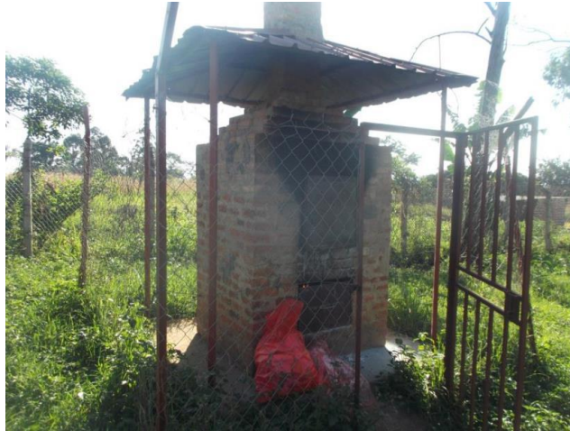
Figure 11: Incinerator at Panyadoli Health Centre IV, Kiryandongo Refugee Settlement in Central Ward in Bweyale Town Council
