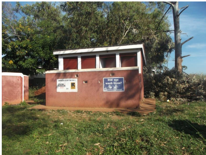
Figure 12: Latrine at Panyadoli Health Centre IV, Kiryandongo Refugee Settlement
