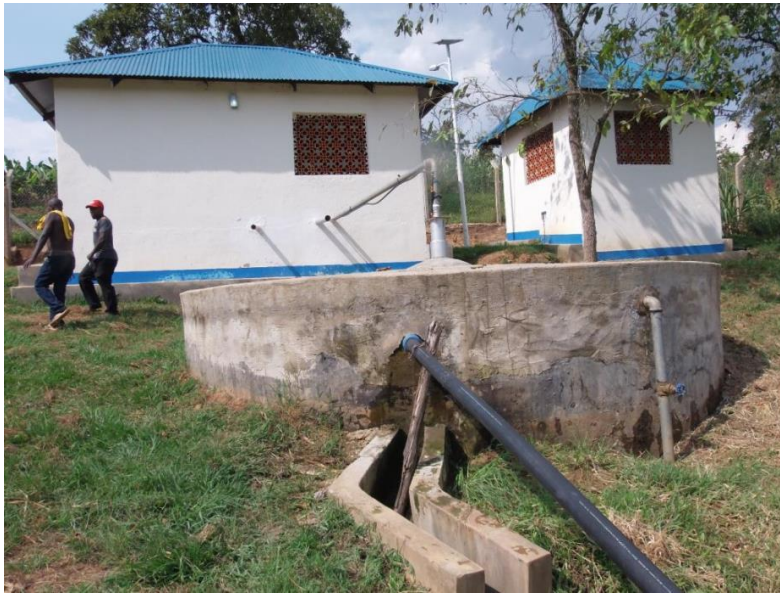
Figure 25: Water treatment tank for gravity water at Kyaka II
