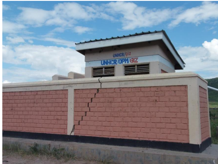
Figure 22: One of the latrines with a damaged superstructure
