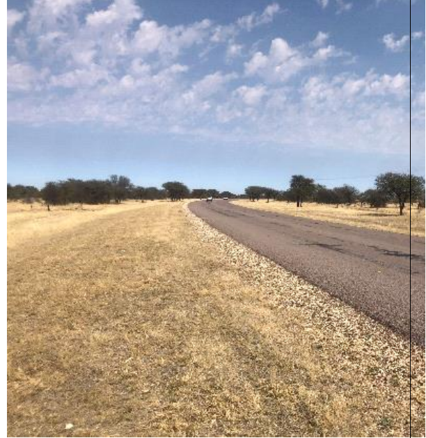
Road reserve between Pitshane Molopo and Mabule for routing of the 66 kV transmission line
