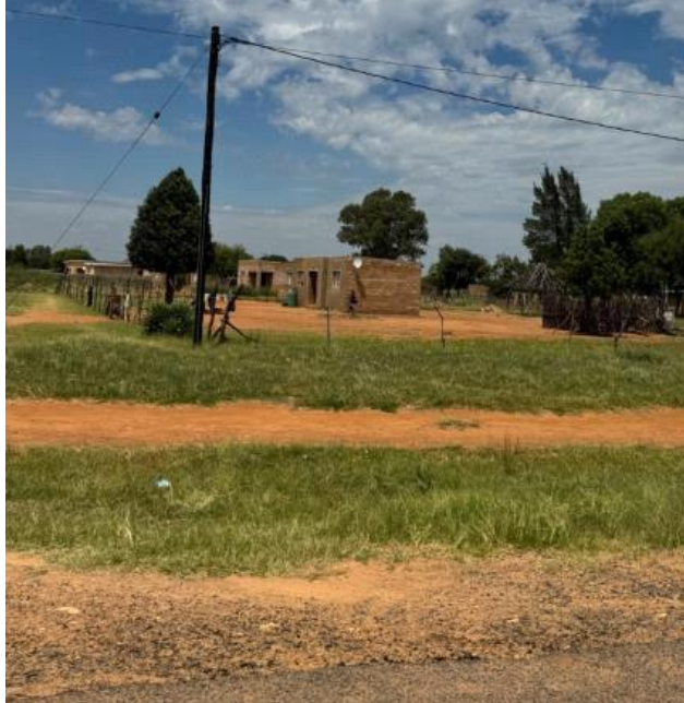
Road reserve in Pitshane Molopo for routing of the 66 kV transmission line
