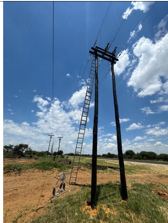
Typical design of a 11kV line structure.
