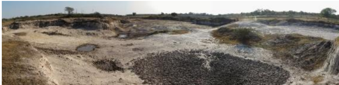
Excavations in wetland areas
