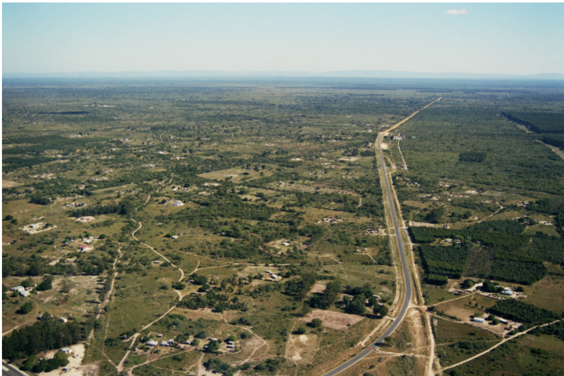
Figure 8 The R22/P444 tared main road in the area of Mbazwana showing the cleared road reserve.
