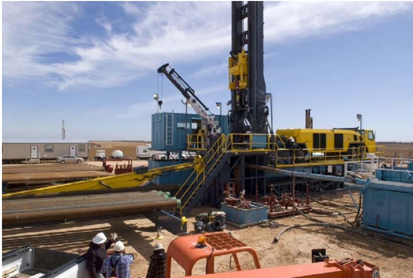
Figure 5 A drill rig that is capable of drilling to depths of 2,000 m to obtain large diameter core and directional drilling techniques. The drill pad setup of an Atlas Copco Predator drill rigs is used as an example. http://multimedia.atlascopco.com/#1452609579665_16
