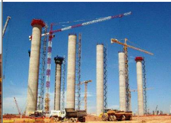
Air cooled condenser columns - Unit 1 January 2010
