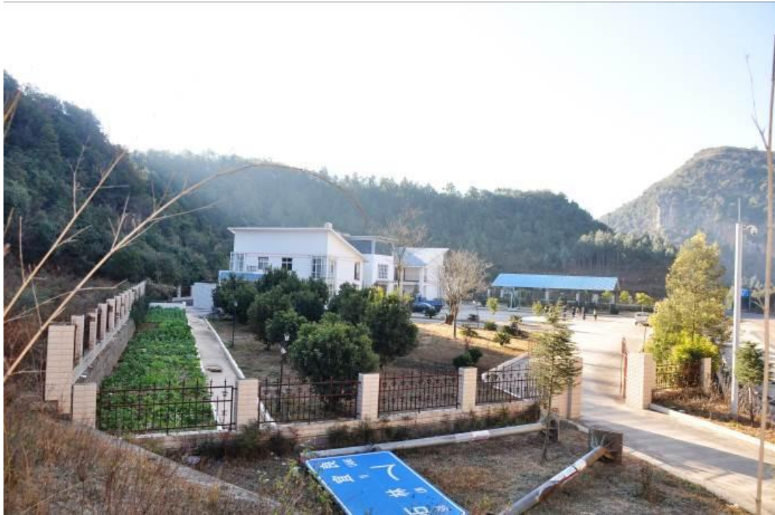
Figure 11 the status of 9 villages office of Yiliang maintenance station
