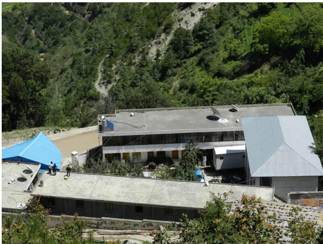
Figure 9 the status of Shusong control station
