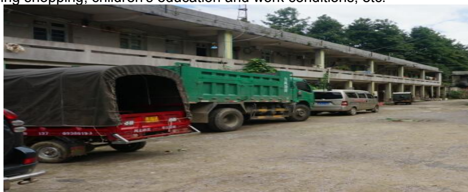
Figure 8 Office Building of the Xinjie Town Highway Management Station
