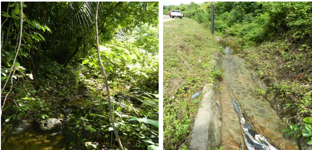
Figure 1.8: North Creek and Road Side Drain with Garbage
