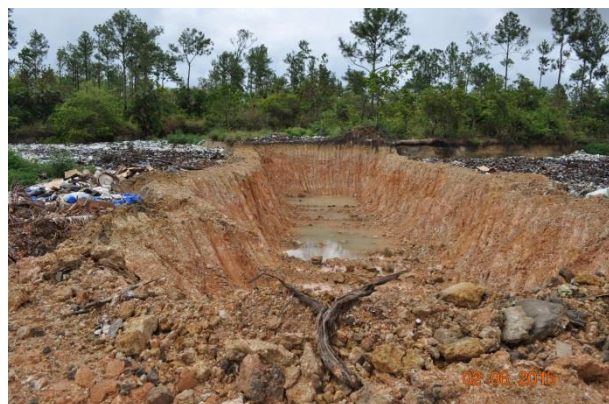
Waste trench – Placencia Dumpsite (area 2). The adjacent trenches are full of trapped water, waste is floating on the surface
